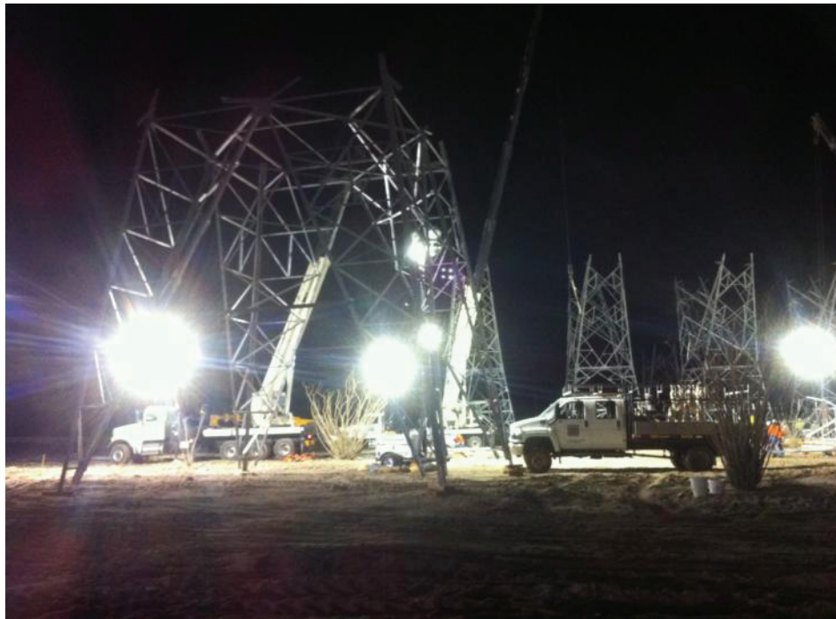
Figure 9: Night work at S2 Yard, Link 1.
