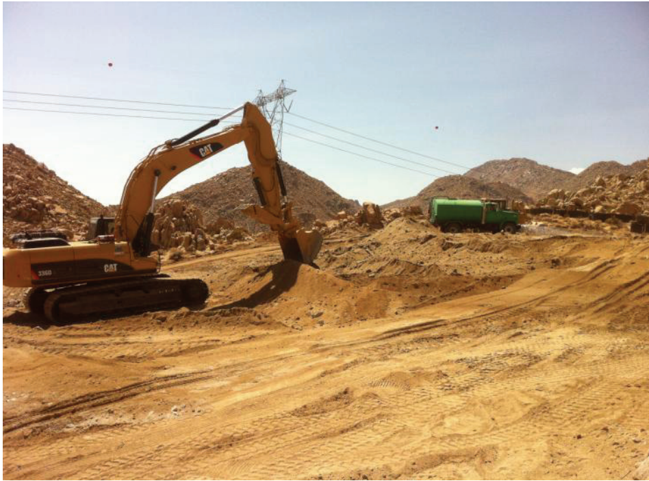
Figure 1: Grading at EP269 pull site, Link 1.
