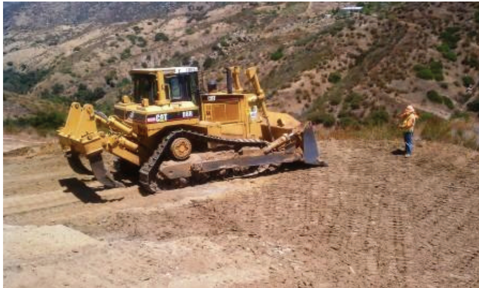
Figure 4: Grading on the Slay property, Link 4.
