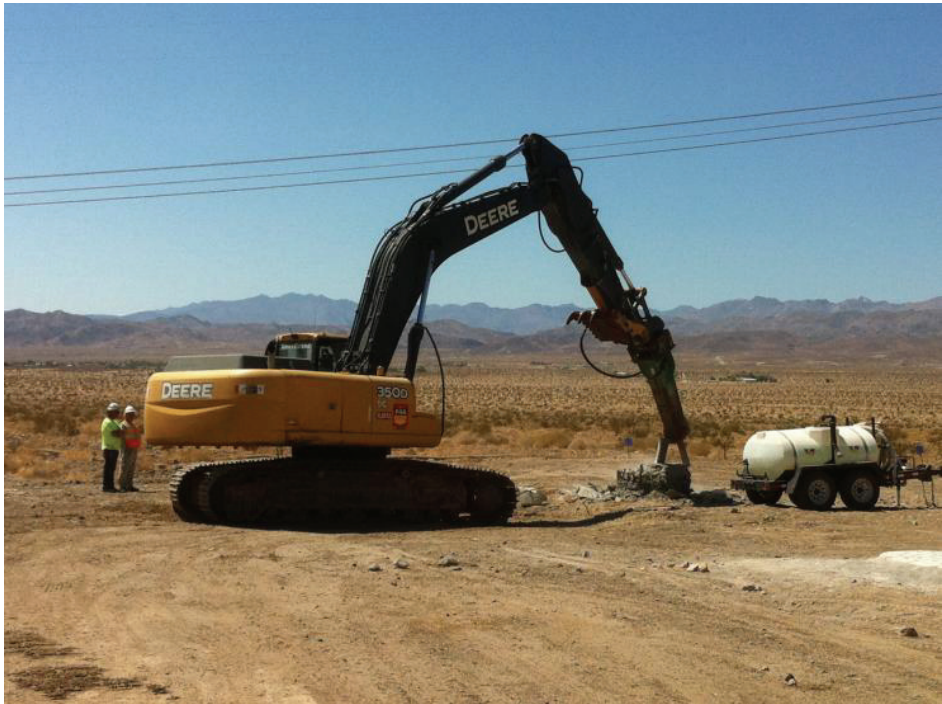
Figure 2: Demolishing foundation reveals at EP303-2, Link 1.
