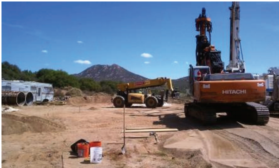
Figure 3: Drilling at EP89, Link 2
