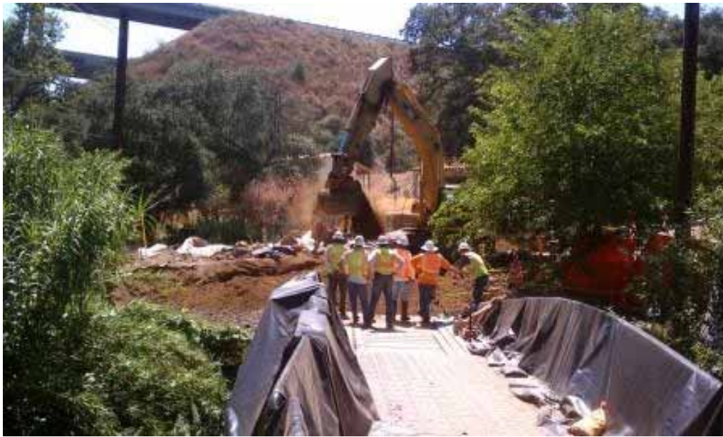
Figure 4: Earthwork being performed on the west side of Bauer Bridge. (Link 4)
