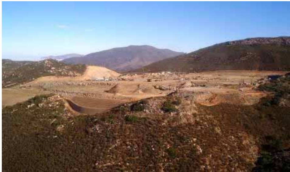
Figure 6: View of Suncrest Substation from the air. (Link 3)
