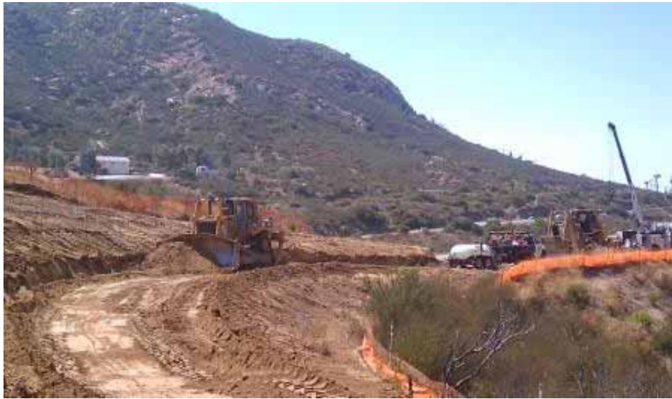
Figure 3: Grading at the Slay Property. (Link 4)
