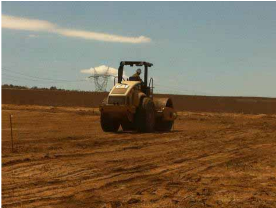
Figure 7: Helicopter pad compaction at AER Yard. (Link 1)
