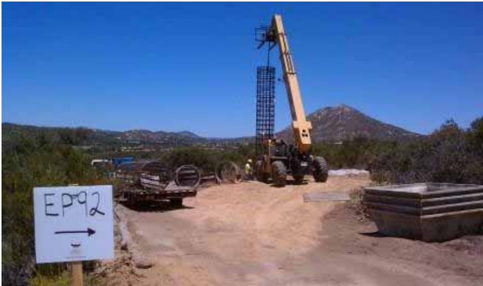
Figure 2: Rebar cages being set at EP92. (Link 2)
