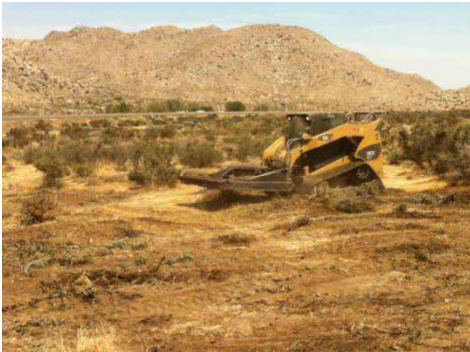
Figure 8: Vegetation clearing at Fromm Yard. (Link 1)
