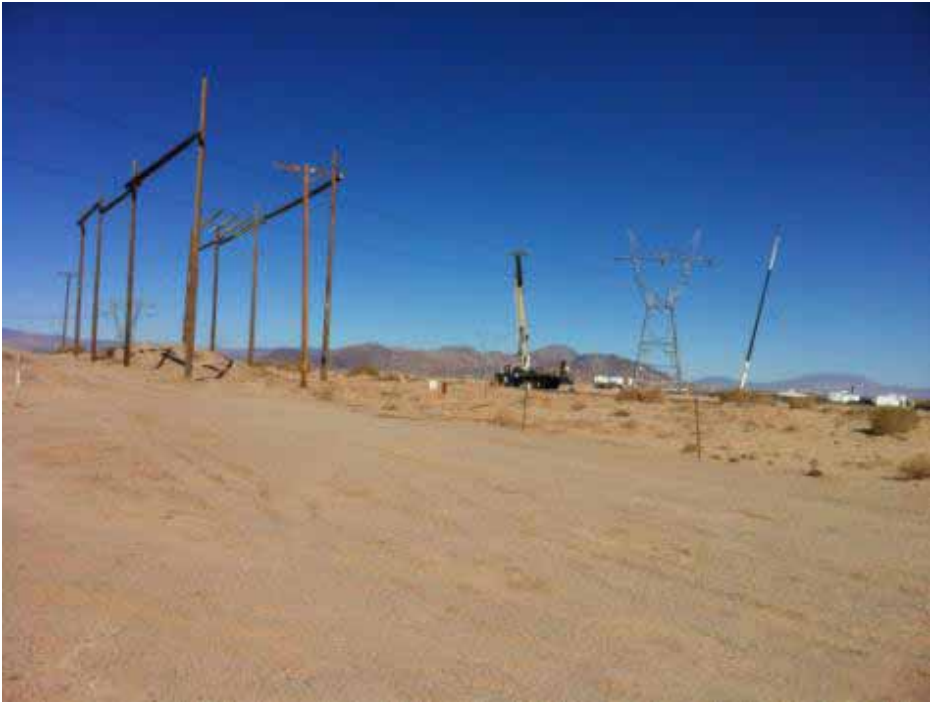
Figure 1: Guard structures near Evan Hewes Highway. (Link 1)
