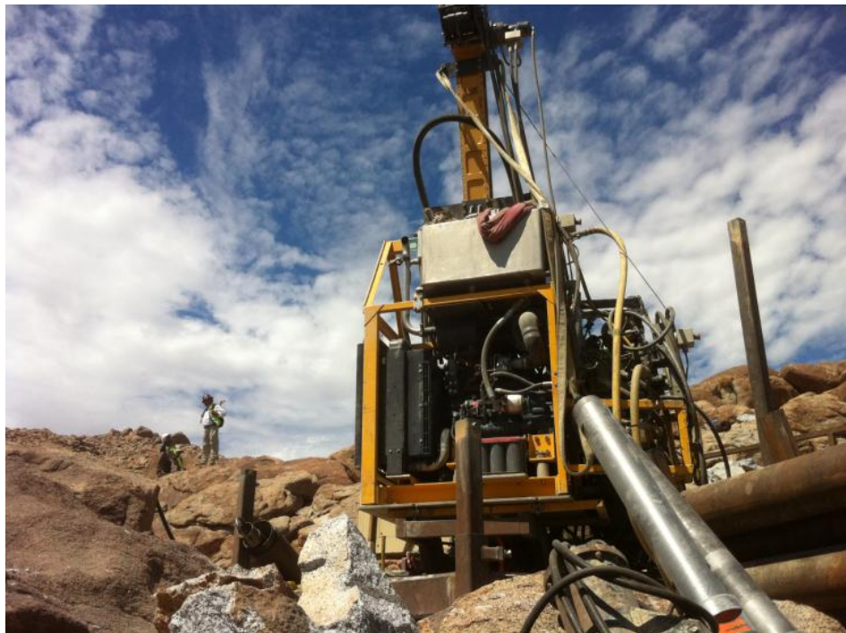
Figure 2: Micropile drilling at EP279-1. (Link 1)
