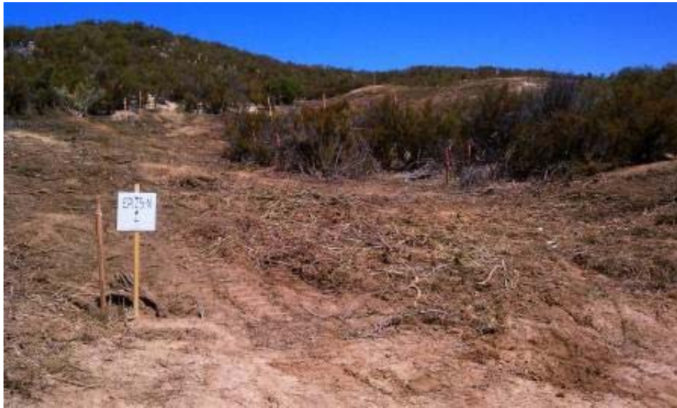
Figure 3: Brush clearing at EP125 pull site. (Link 2)
