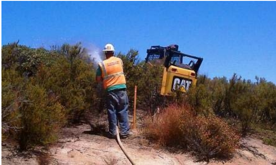
Figure 4: Brush clearing with watering on USFS lands. (Link 2)
