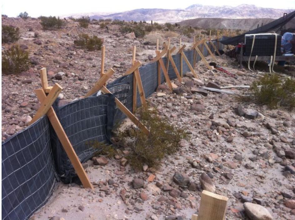
Figure 5: Example of gecko exclusionary fencing (installed at EP280-2). (Link 1)
