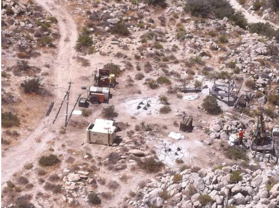
Figure 1: Micropile drilling at EP259B. (Link 1)
