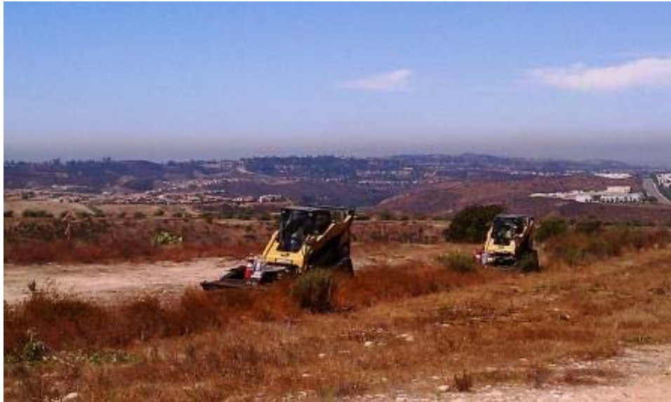
Figure 8: Brush clearing at Sycamore Construction Yard. (Link 5)
