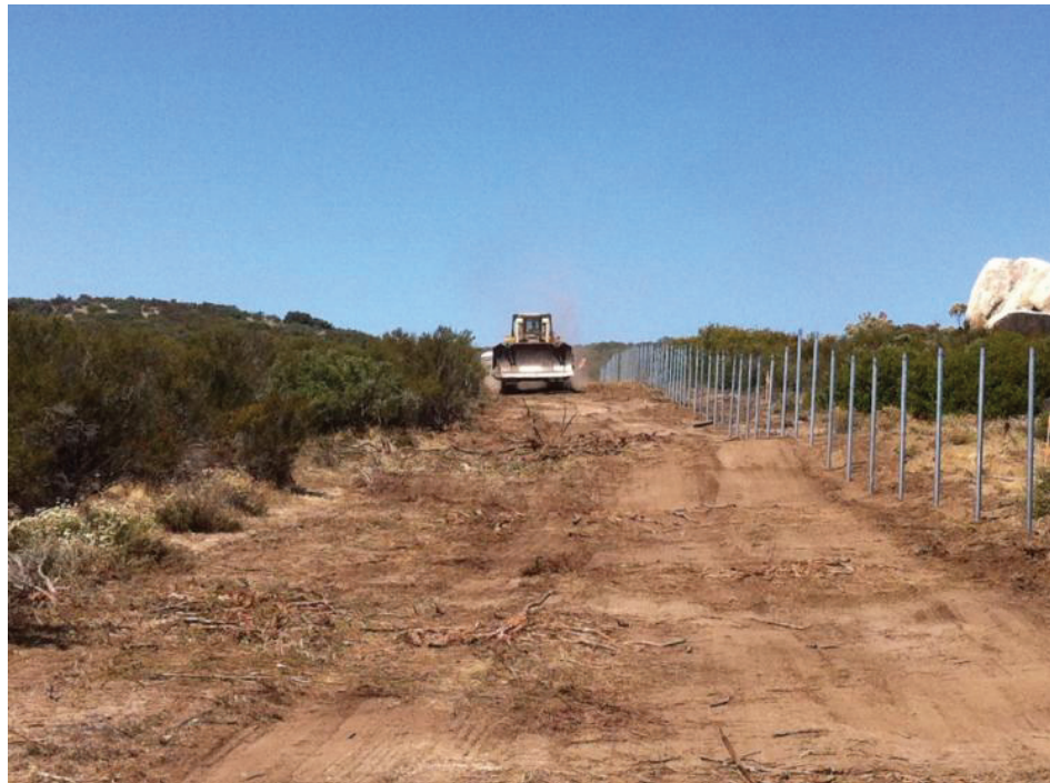
Figure 12: Vegetation clearing and fence installation at McCain Valley Yard. ( Link 1 )
