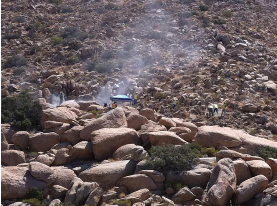
Figure 1: Breaking boulders and site preparation work at EP261-1. (Link 1)
