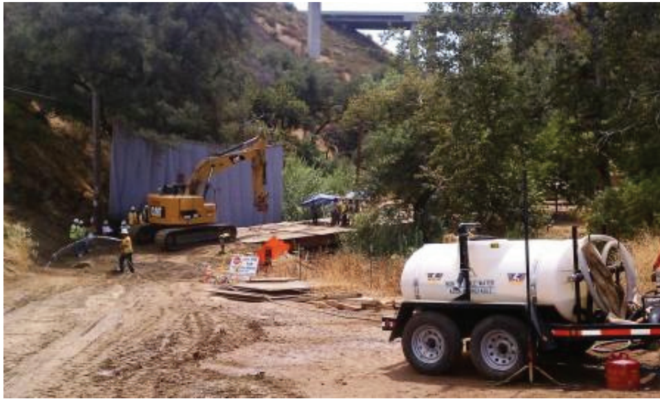
Figure 9: Metal plates being placed on temporary bridge at Bauer Bridge. (Link 4)
