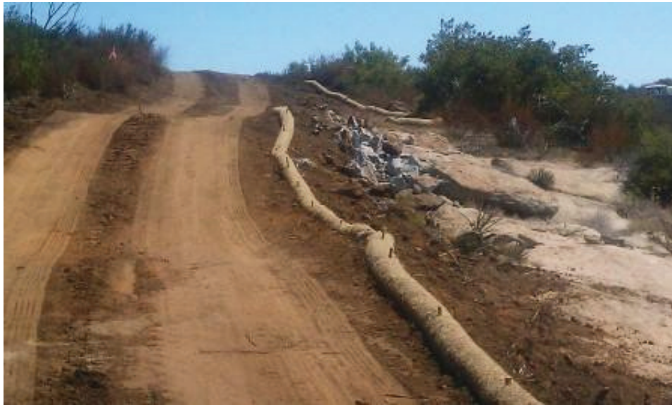
Figure 3: BMPs on newly graded access road to EP39. (Link 2)
