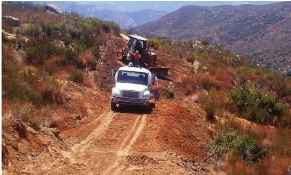
Figure 4: Grading operations on access road to EP40-1. (Link 2)
