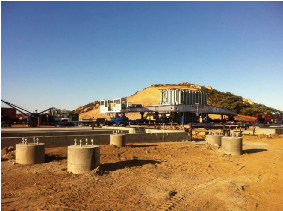
Figure 11: Delivery of the first transformer at Suncrest Substation. ( Link 3 )
