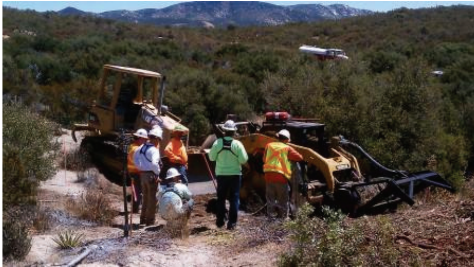
Figure 7: Vegetation clearing on USFS lands near EP126-1. (Link 2)
