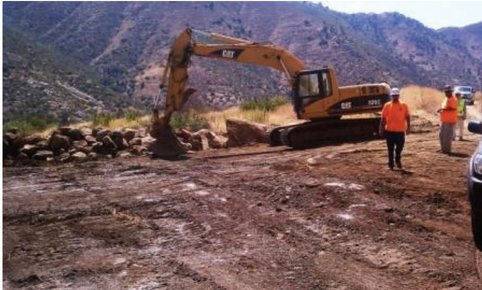
Figure 10: Grading and boulder removal on access road to CP70-3. (Link 5)
