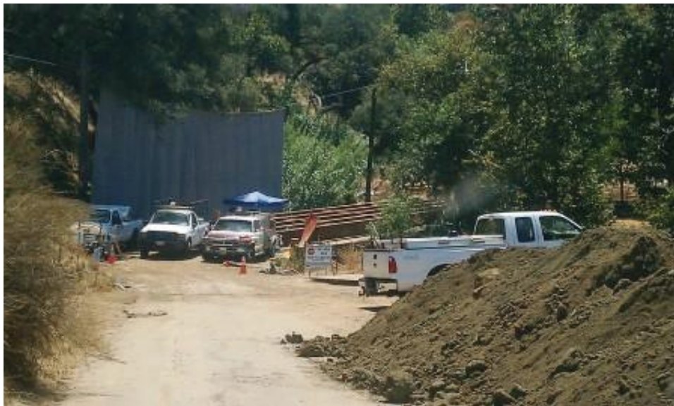
Figure 8: Temporary bridge installation at Bauer Bridge. (Link 4)
