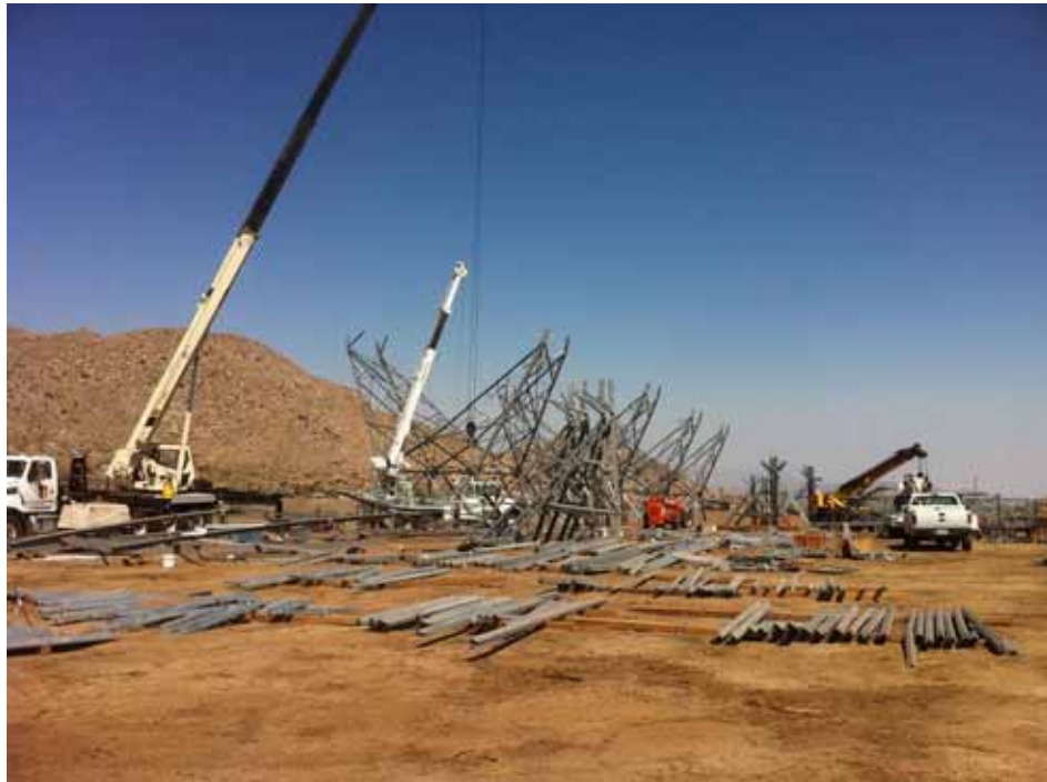
Figure 10: Steel assembly at Fromm Yard. (Link 1)
