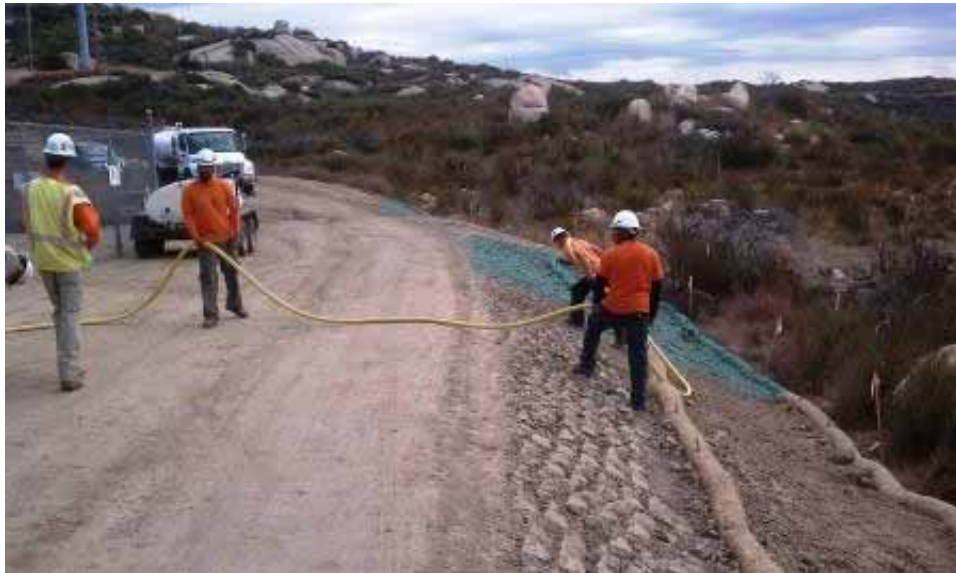
Figure 8: Hydromulching slopes on access road to Barrett Construction Yard near Barrett substation. (Link 2)
