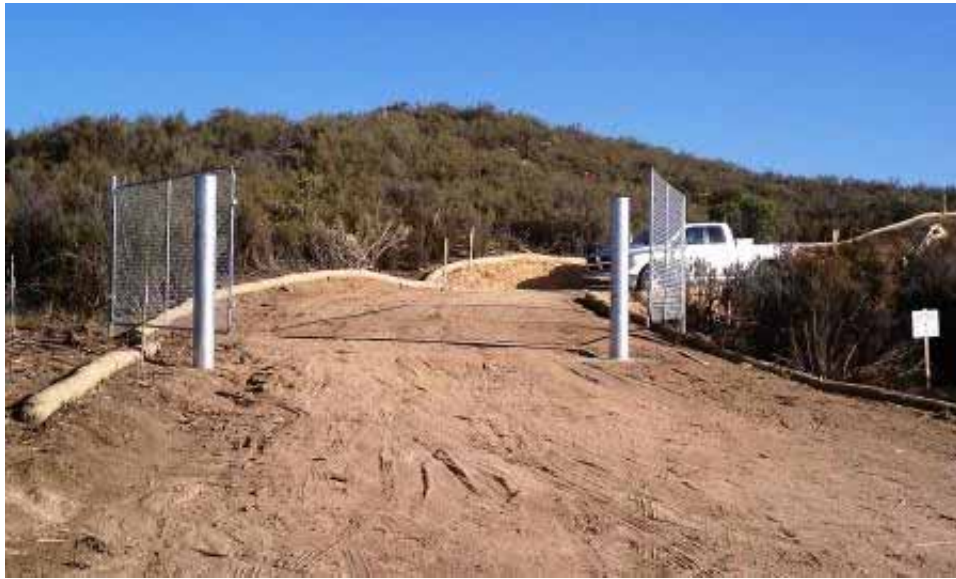
Figure 3: Permanent gate installation at EP126-1. (Link 2)
