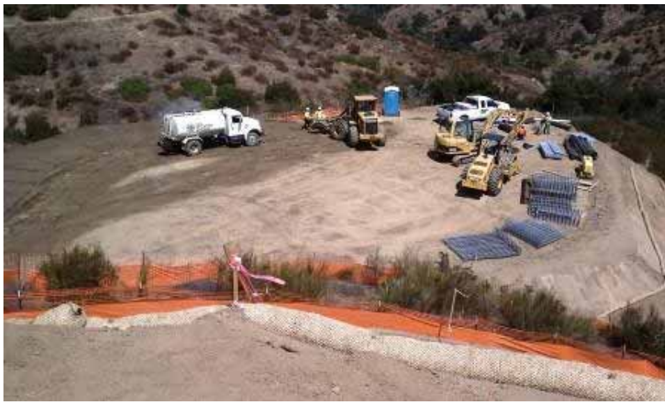
Figure 4: Grading of pad for CP87-1 and CP88-1. (Links 4 & 5)
