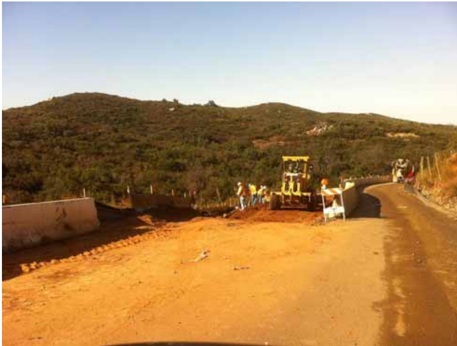
Figure 9: Construction of the soil retention wall along BBTT. (Link 3)
