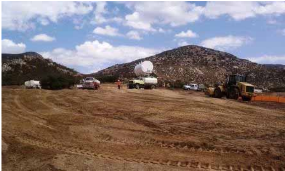
Figure 11: Grading pull site at Thing Valley Yard. (Link 5)
