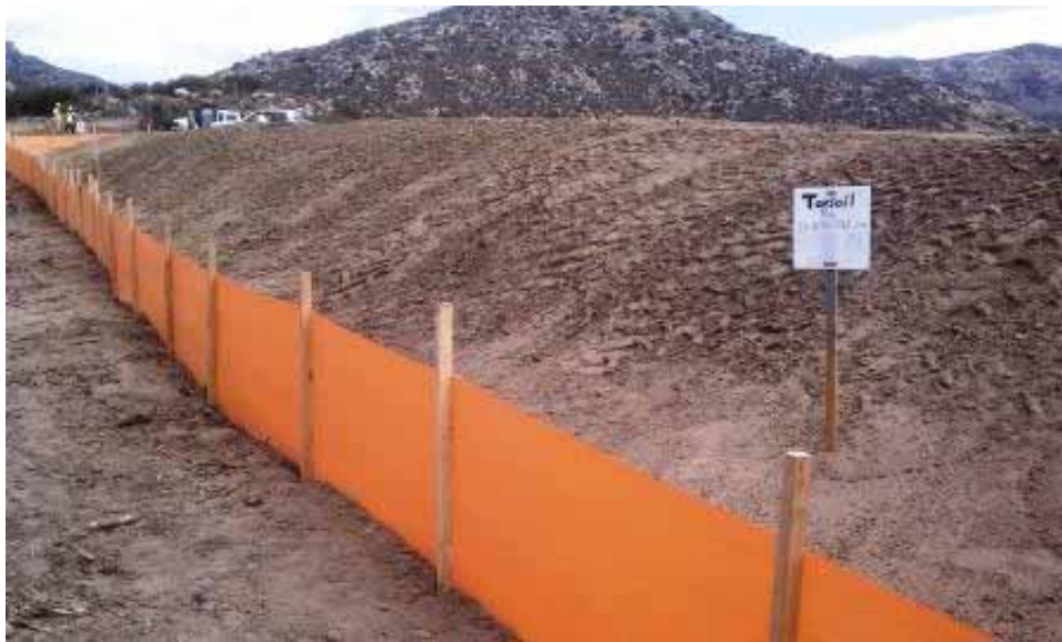
Figure 12: Topsoil stockpiled at Thing Valley Yard. (Link 2)
