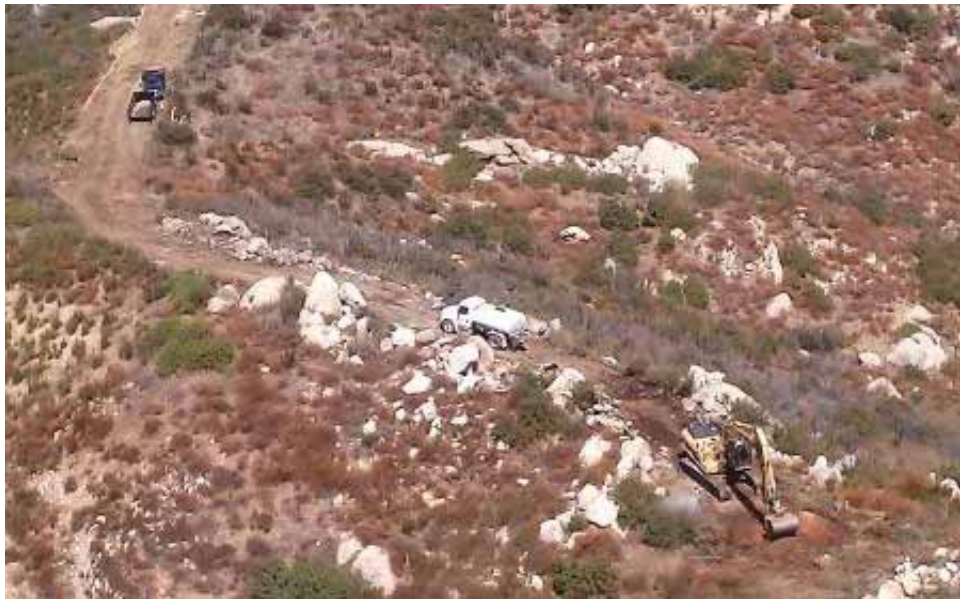
Figure 2: Clearing for access road to Barrett Construction Yard. (Link 2)
