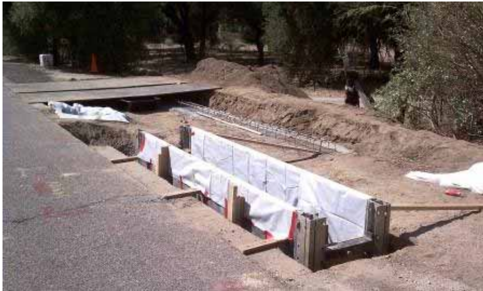
Figure 7: Driveway construction for CP64/65 pull site. (Link 5)
