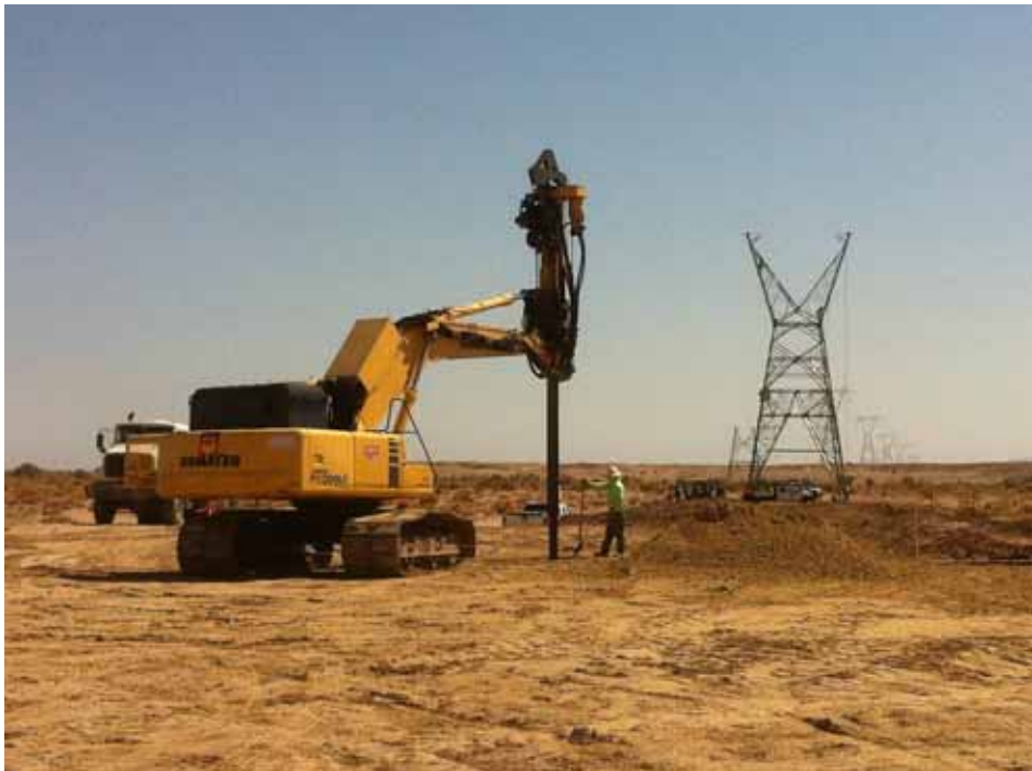
Figure 1: Drilling snubs at the EP322/323 pull site. (Link 1)
