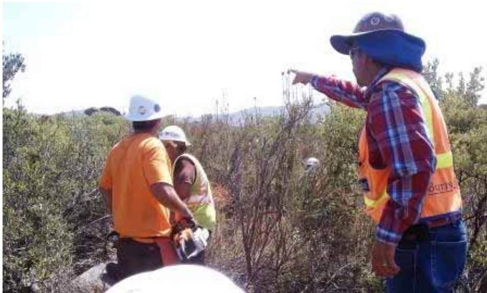
Figure 5: Vegetation clearing on access road to CP98-1. (Link 2)
