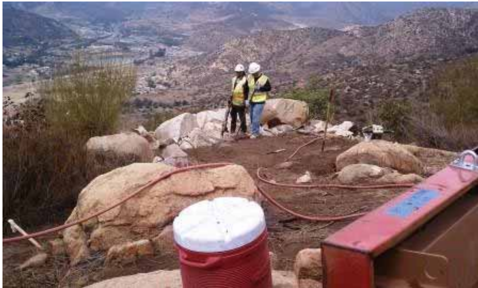
Figure 5: Boulder removal and site preparation at CP47-2. (Link 5)
