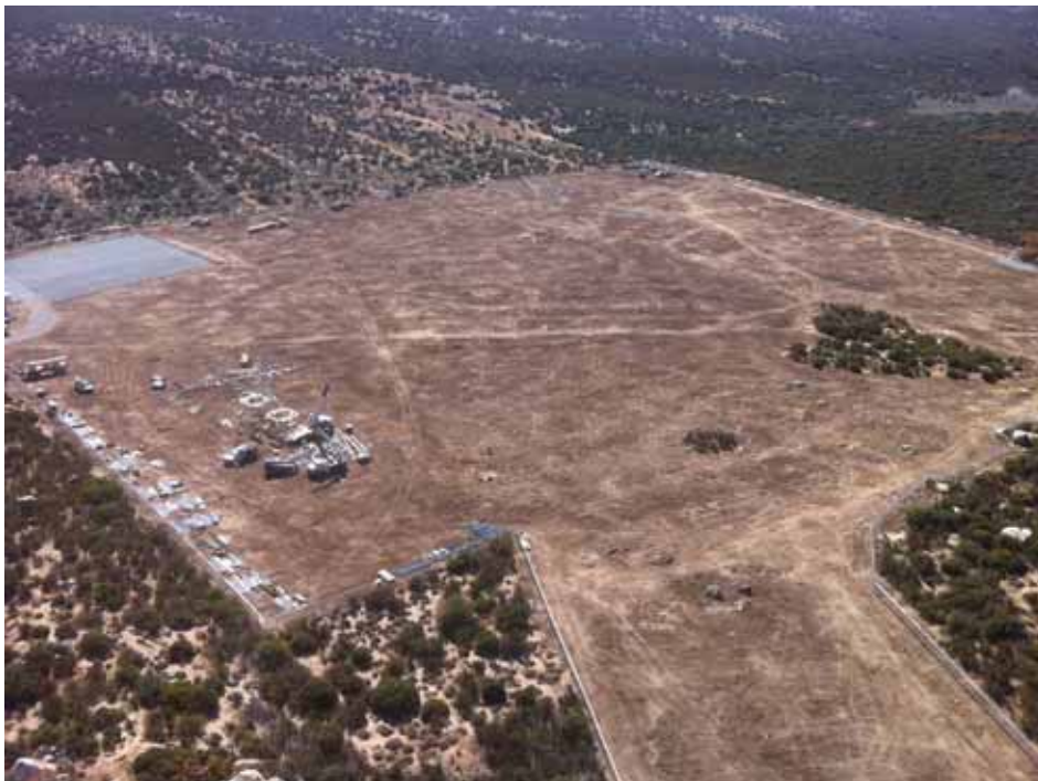
Figure 10: Aerial view of McCain Valley Construction Yard. (Link 1)
