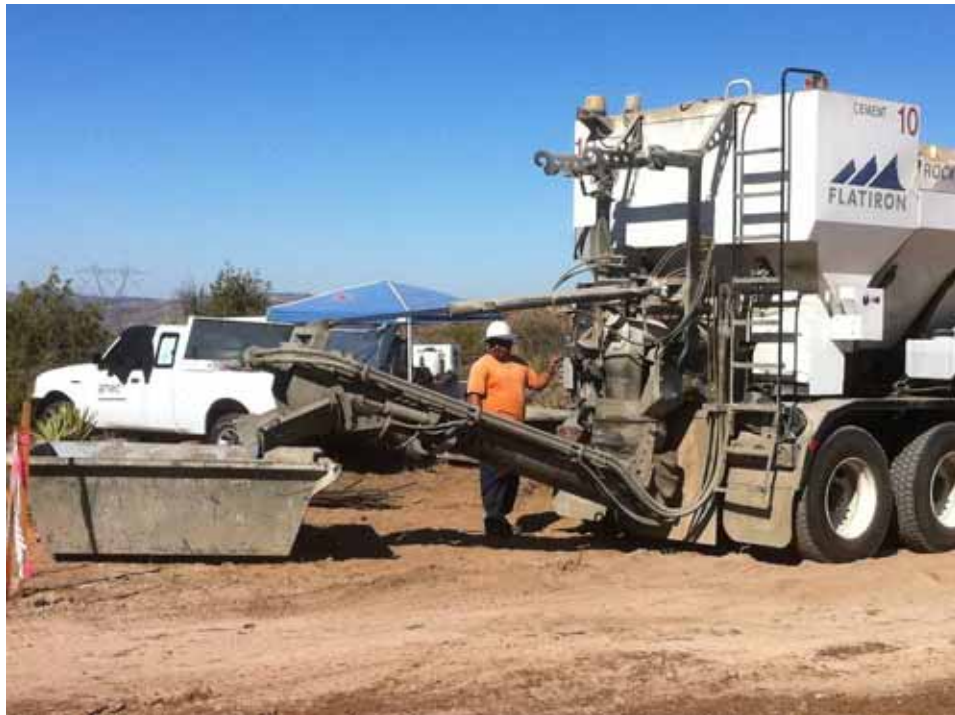
Figure 1: Using an eco-pan for concrete truck washout at EP251. (Link 1)
