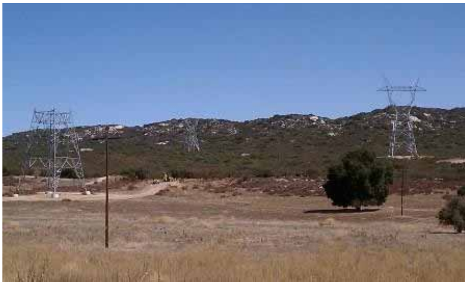
Figure 2: View of towers EP90 (left), EP91 (right), and EP92 (middle). (Link 2)
