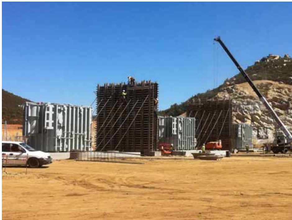
Figure 9: Forming blast walls between transformers at Suncrest Substation. (Link 3)
