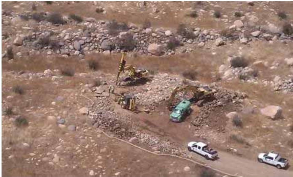
Figure 7: Conventional drilling in a rocky area at CP70-3. (Link 2)
