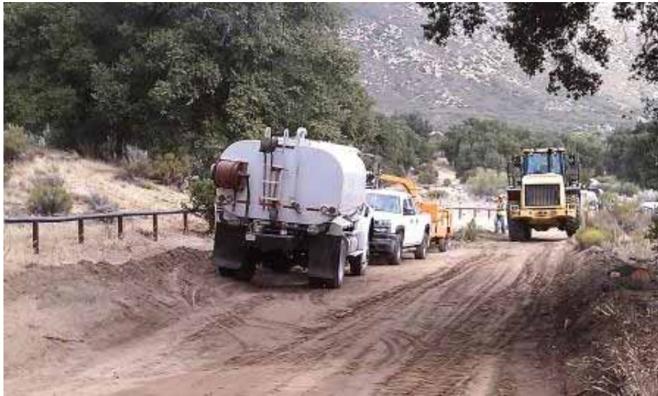
Figure 3: Road improvement on La Posta Road. (Link 2)
