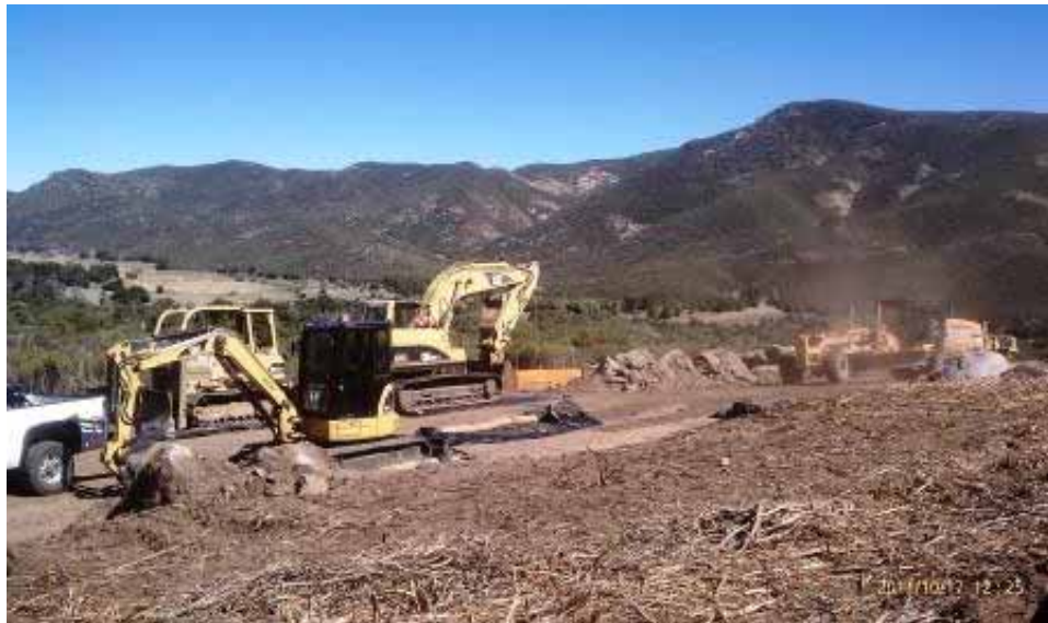
Figure 6: EP141 pull site with BMPs in background. (Link 2)
