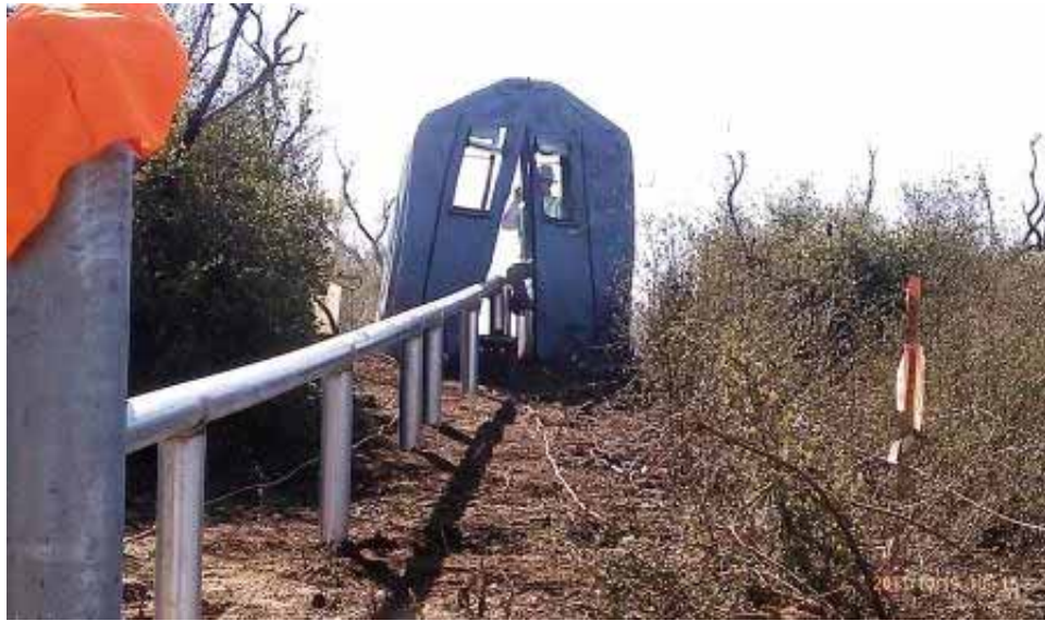
Figure 5: Welding fence along access road to Barrett Construction Yard. (Link 2)
