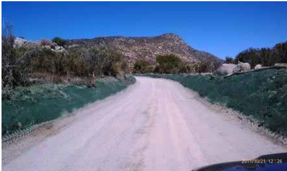
Figure 10: Hydromulching with green indicator ink along La Posta Road. (Link 2)
