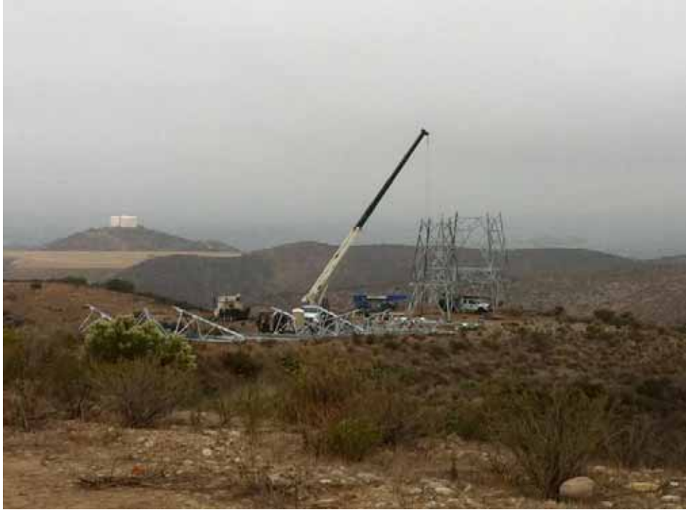
Figure 14: Tower assembly at Sycamore Yard. (Link 5)
