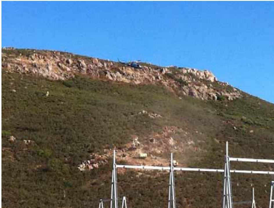
Figure 9: Micropile work at CP109. (Link 5)
