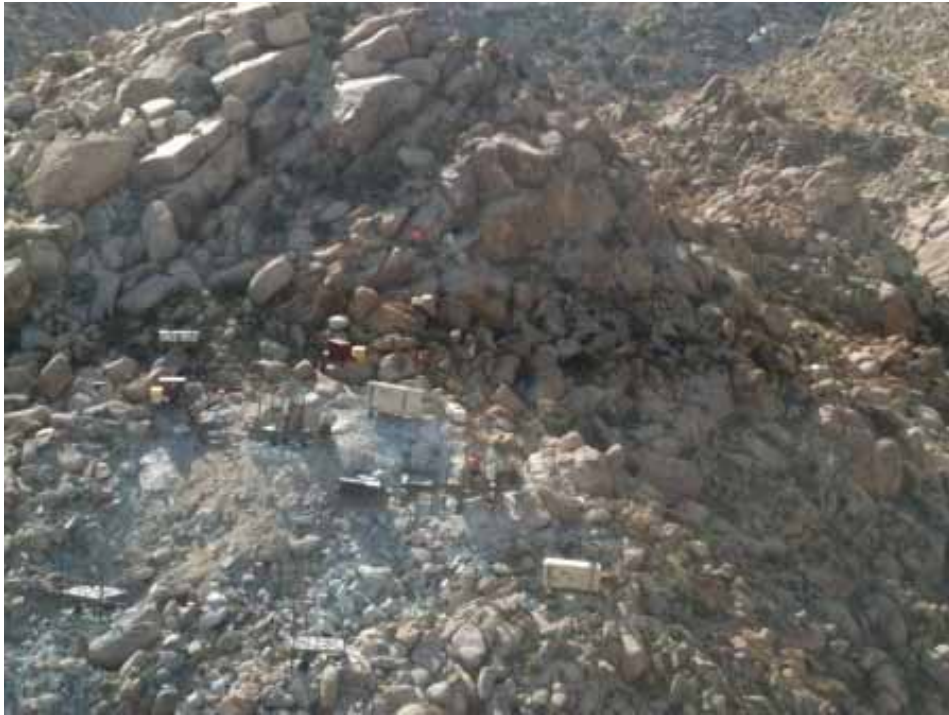
Figure 1: Micropile drilling at EP267-2. ( Link 1 )
