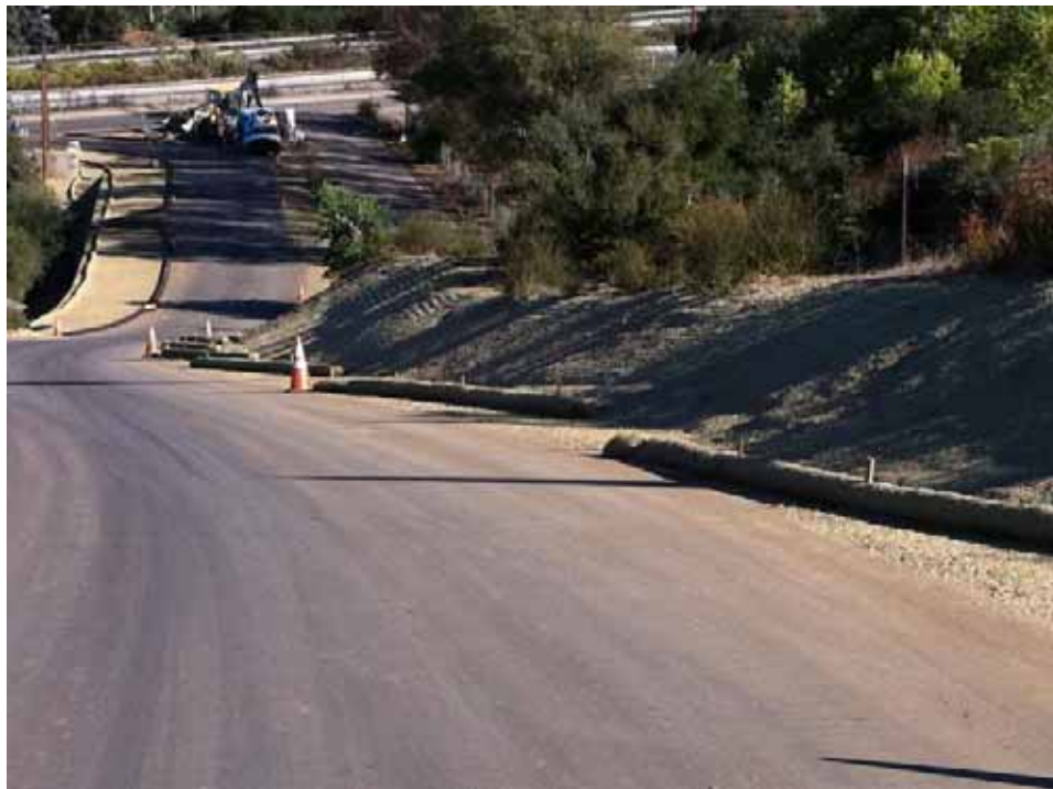
Figure 11: Hydromulching along access road to CP100-1. (Link 5)
