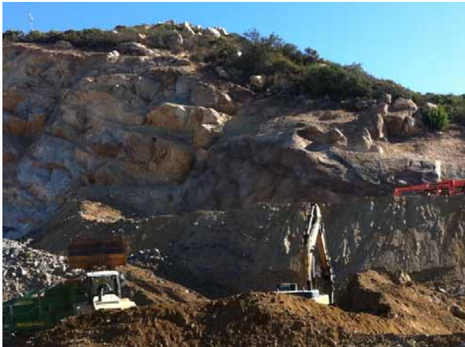
Figure 12: Acid wash application to soil nail wall. (Link 3)
