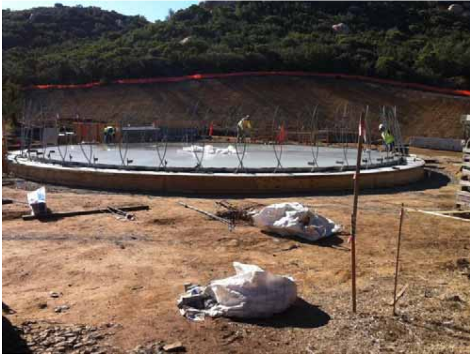
Figure 13: Water tank foundation near trailers at Suncrest Substation. (Link 3)
