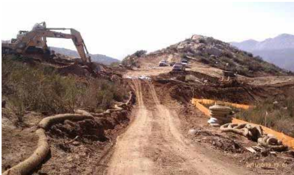
Figure 4: Access road to Barrett Construction Yard. (Link 2)
