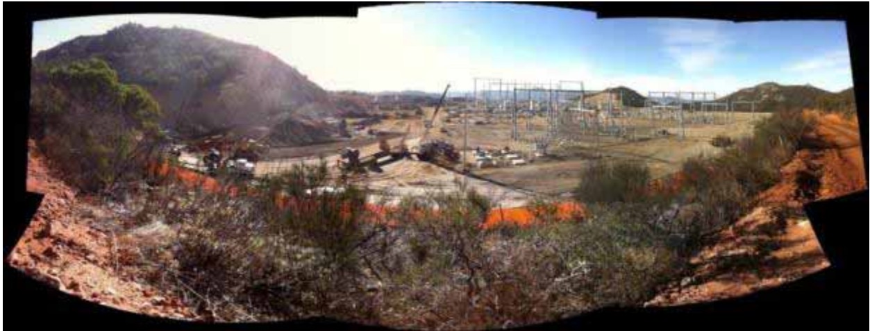
Figure 10: Panoramic view of Suncrest Substation. (Link 3)
