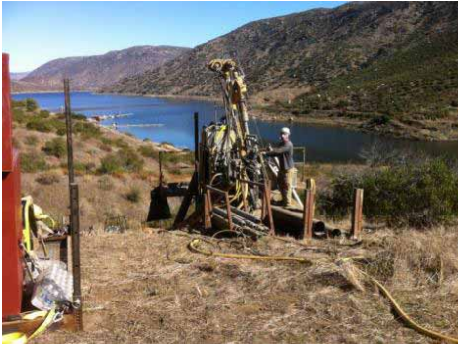
Figure 6: Micropile drilling at CP81-1. (Link 5)
