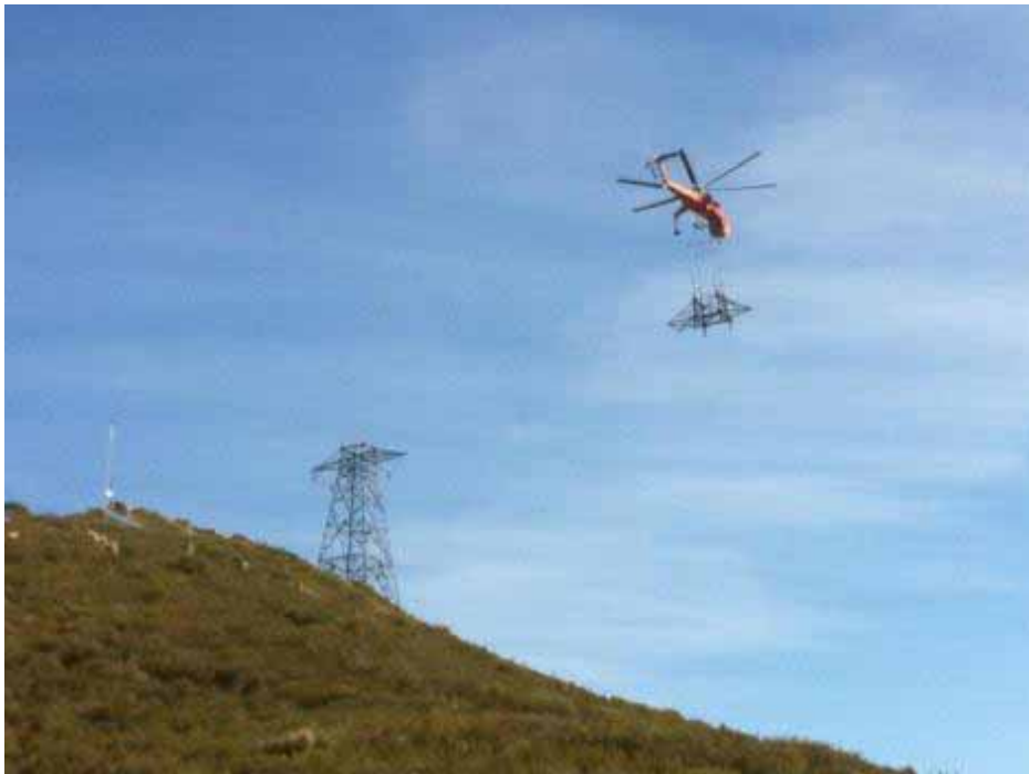
Figure 7: Aircrane setting bridge at CP107. (Link 5)
