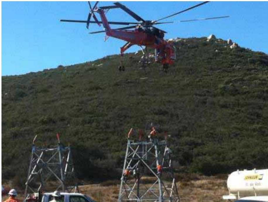
Figure 8: Aircrane getting ready to pick a tower at Wilson Yard. (Link 3)
