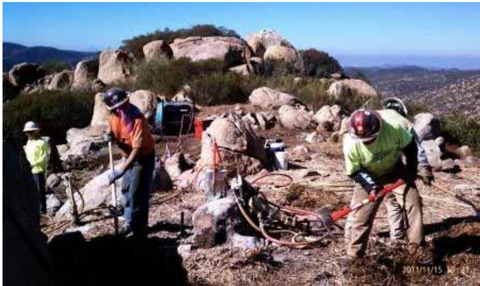
Figure 2: Brush clearing/boulder busting crew at EP6-1 TSAP. (Link 2)
