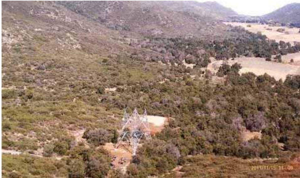
Figure 4: Helicopter view looking north to Tower EP141 and pull site. (Link 2)
