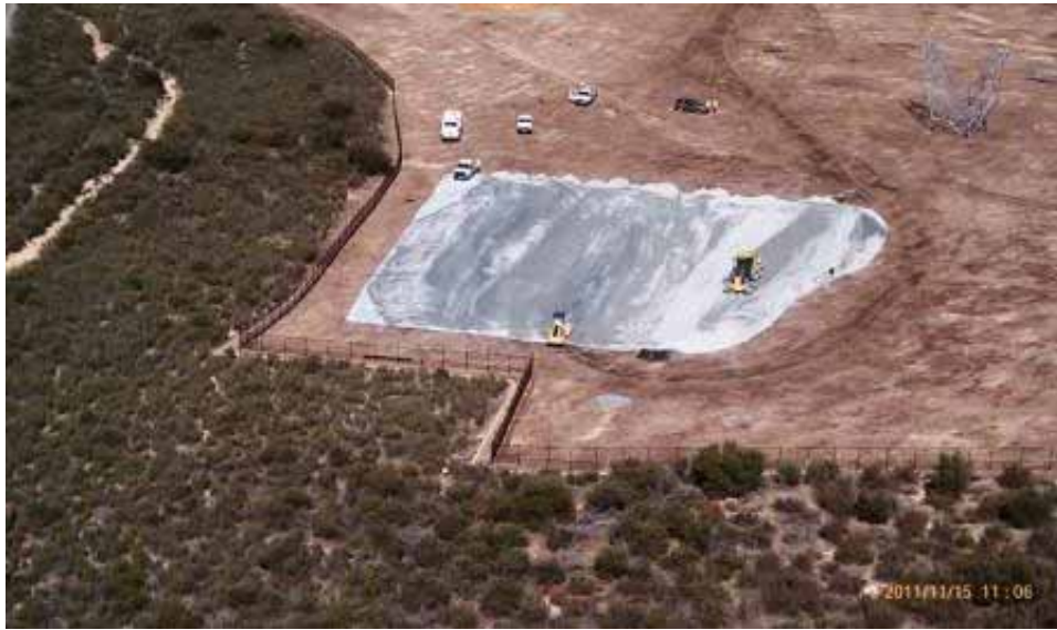
Figure 11: Helicopter pad construction at Thing Valley Construction Yard. (Link 2)
