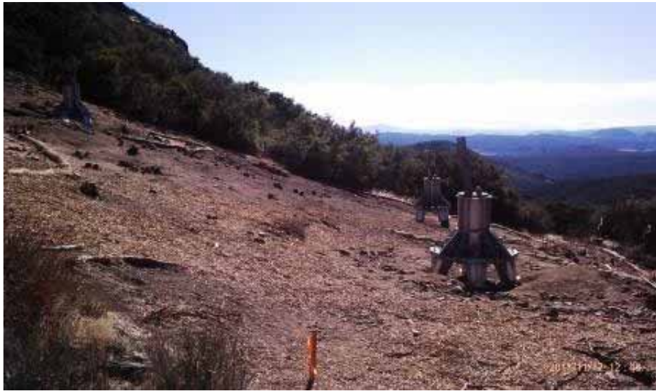
Figure 3: EP140-1 with micropile caps installed. (Link 2)
