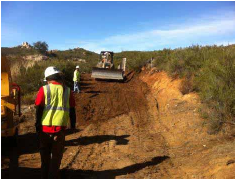
Figure 5: Grading access road to CP106-1. (Link 5)
