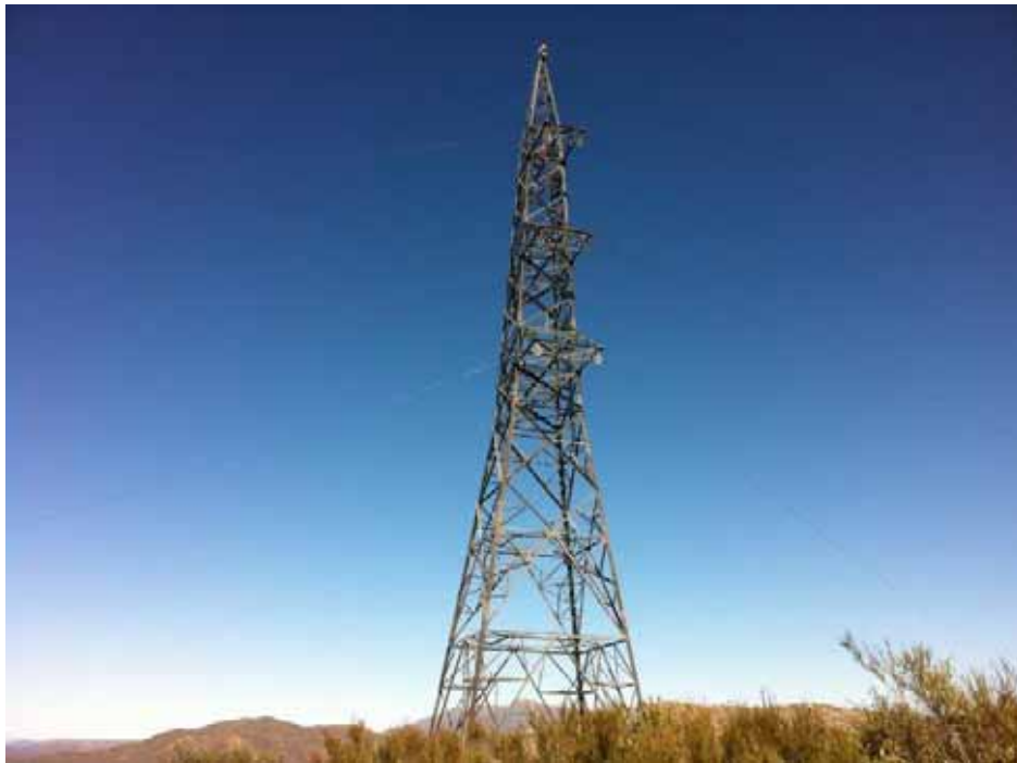
Figure 9: Sock line pulled through CP106-1. (Link 5)
