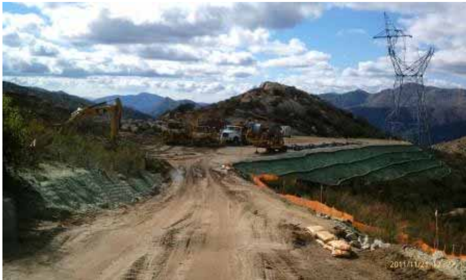
Figure 4: EP47-2 and pull site; tower is under construction. (Link 2)
