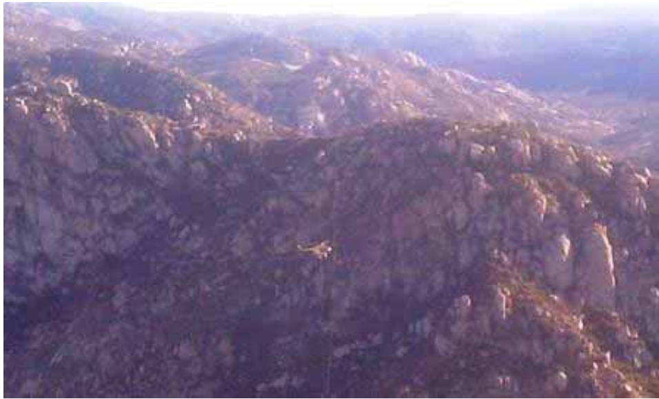
Figure 3: Helicopter running sock line over the mile span from EP43 to EP42. (Link 2)
