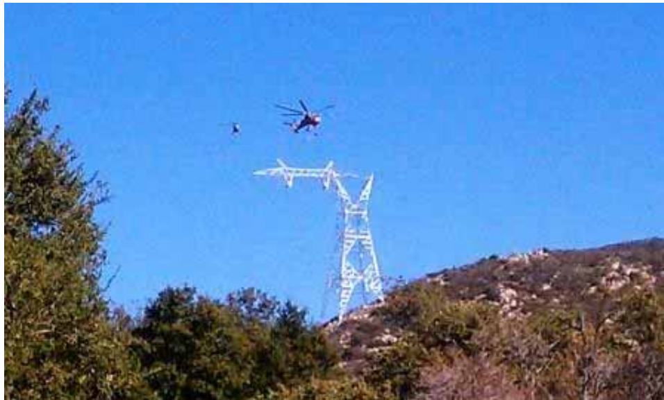
Figure 6: Air crane attempting to set top on tower EP 137.
