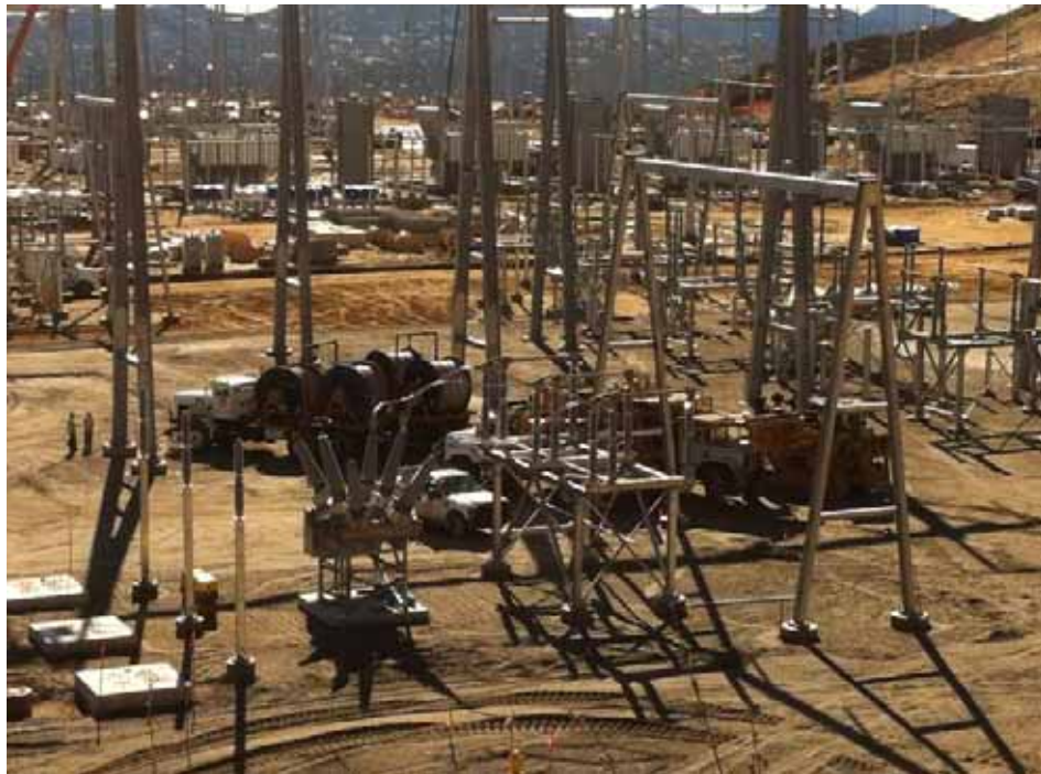
Figure 11: Wire stringing equipment on the Suncrest Substation pad. (Link 3)
