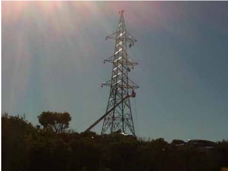
Figure 8: Wire stringing activities at CP100-1. (Link 5)
