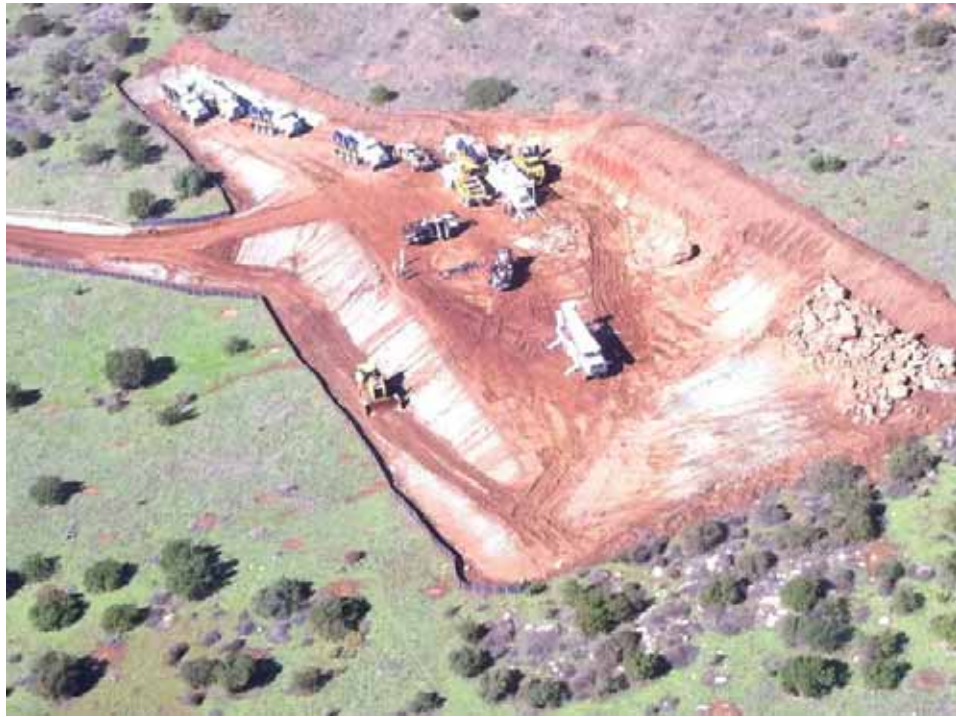
Figure 7: CP55/CP56-1 pull site activities. (Link 5)
