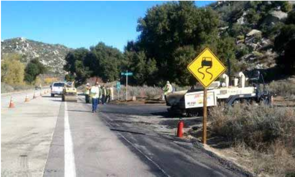
Figure 1: Driveway construction at Cameron Truck Trail & Old Highway 80. (Link 2)
