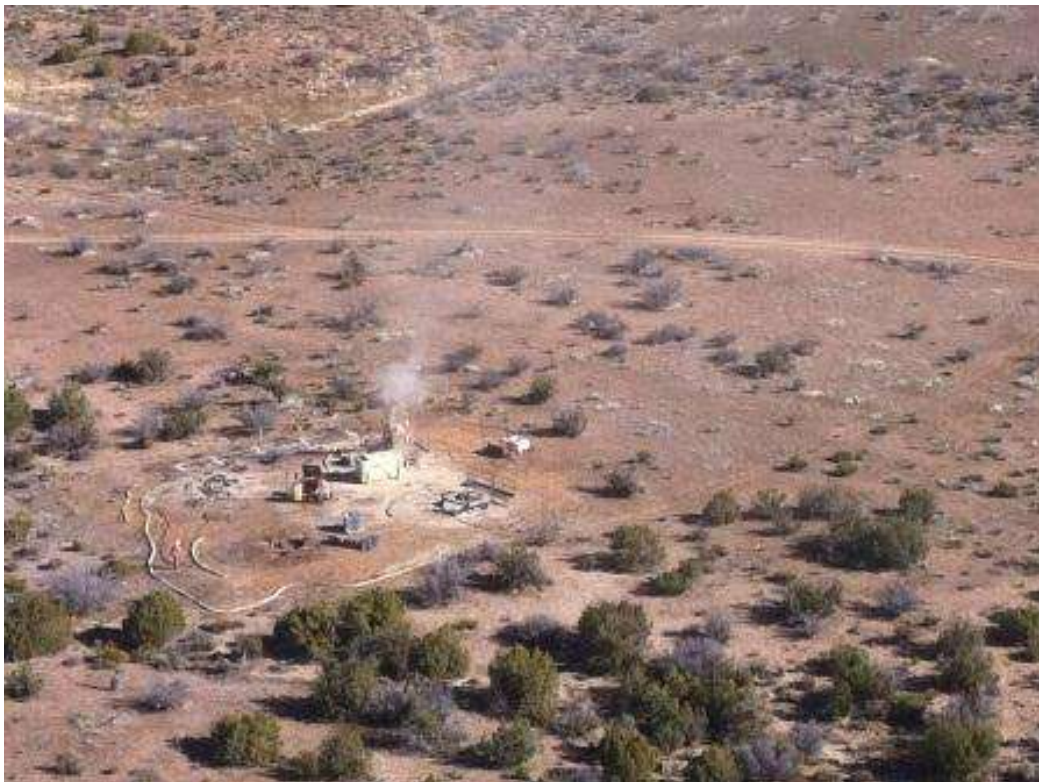
Figure 2: Micropile drilling at EP234-1. (Link 1)
