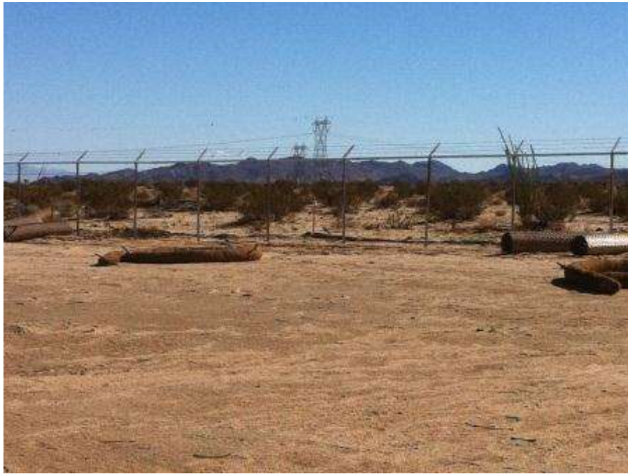
Figure 11: Start of fence removal at S-2 Yard. (Link 1)
