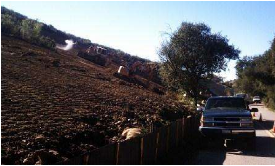
Figure 5: Slope restoration at CP23 pull site. (Link 5)
