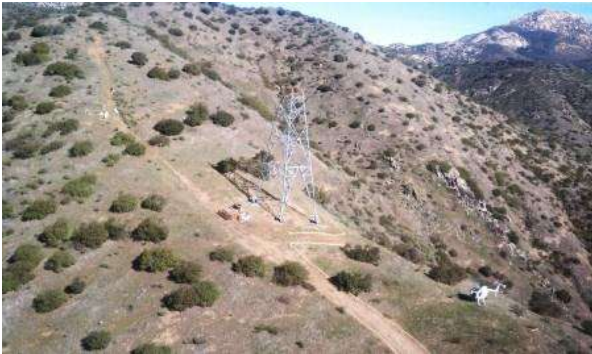
Figure 9: Helicopter noted to be outside of an approved TSAP near CP59.
