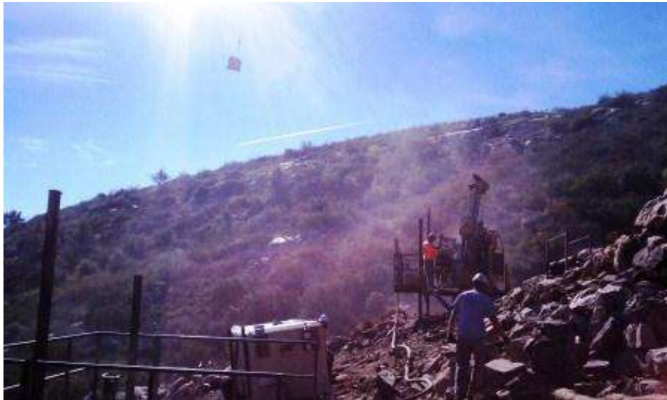
Figure 6: Micropile drilling and incoming helicopter load at CP32-2. (Link 5)
