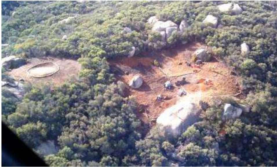
Figure 3: Boulder busting crews prepping site at EP13-3. (Link 2)
