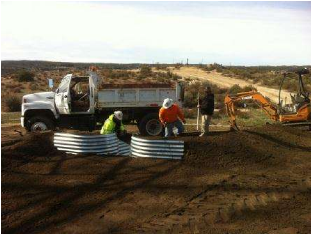
Figure 1: Final grading of the permanent maintenance pad at EP207. (Link 1)
