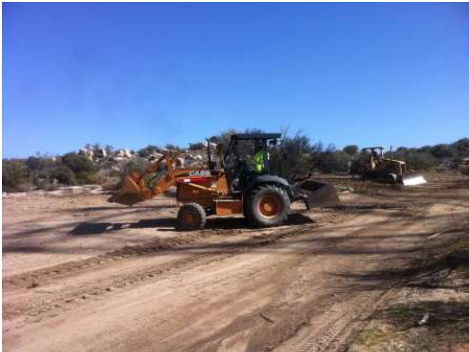
Figure 1: Final grading at Tower EP219-1-E. (Link 1)
