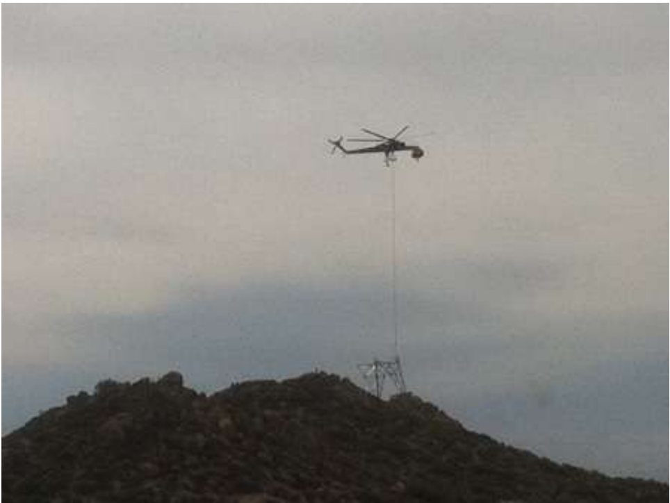
Figure 2: Skycrane assembly at Tower EP234-1. (Link 1)
