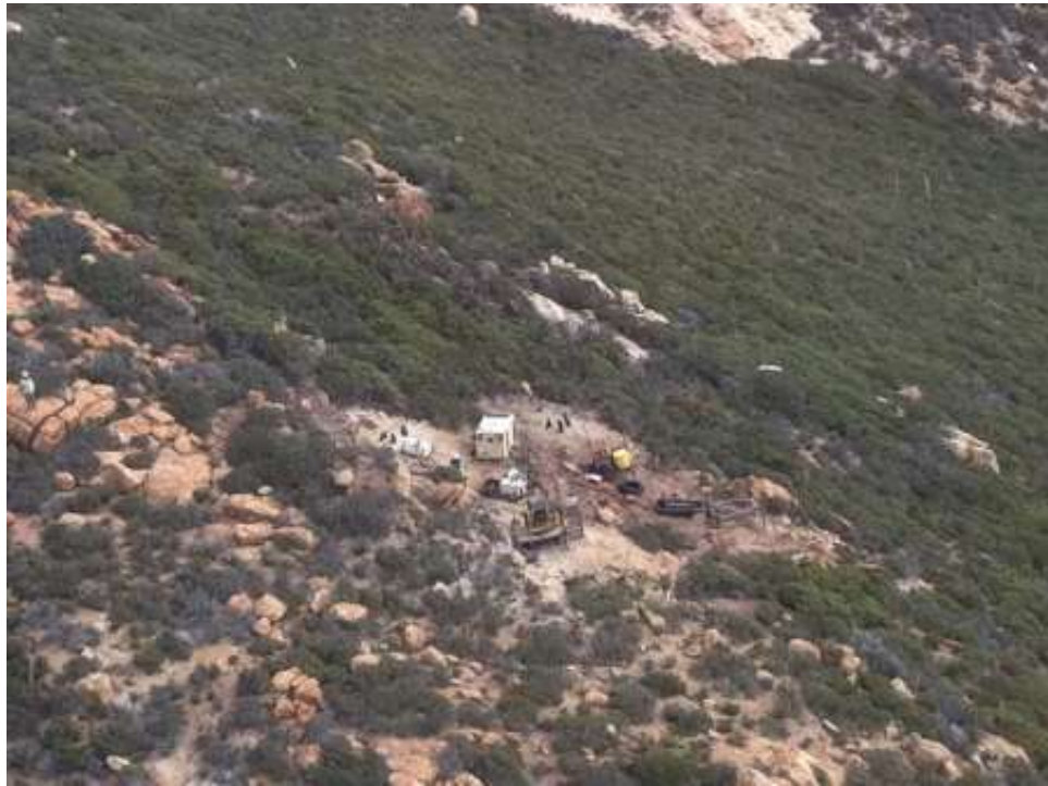
Figure 3: Micropile drilling at Tower EP148. ( Link 1 )
