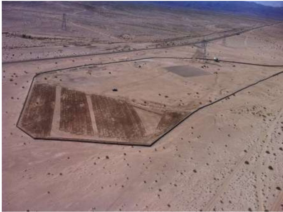
Figure 7: Restoration work occurring in the Plaster City Yard. (Link 1)
