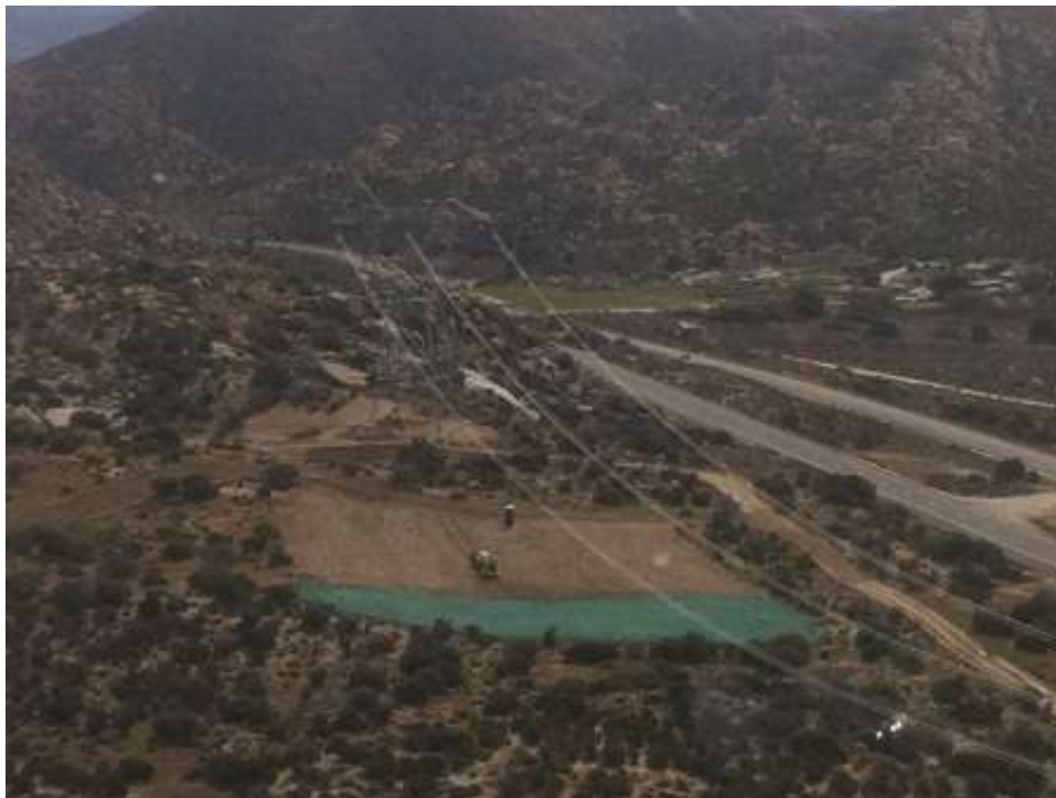
Figure 4: Hydromulching EP219-1 pull site west. (Link 1)
