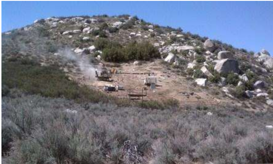
Figure 2: Micropile drilling at EP114-2. ( Link 2 )
