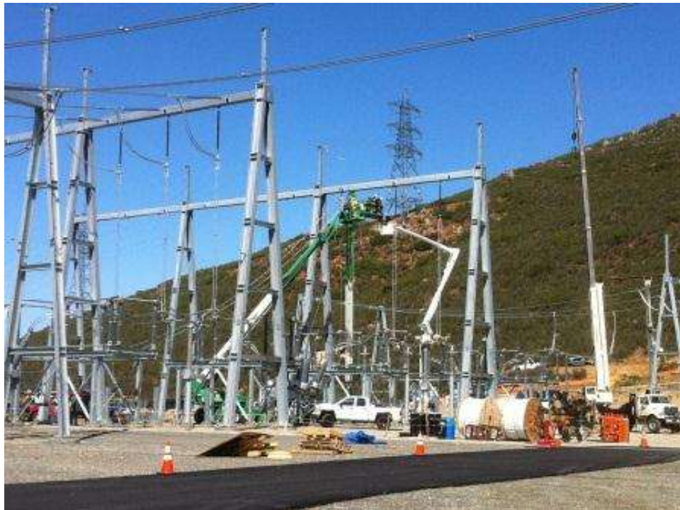
Figure 10: Steel work at Suncrest Substation. (Link 3)
