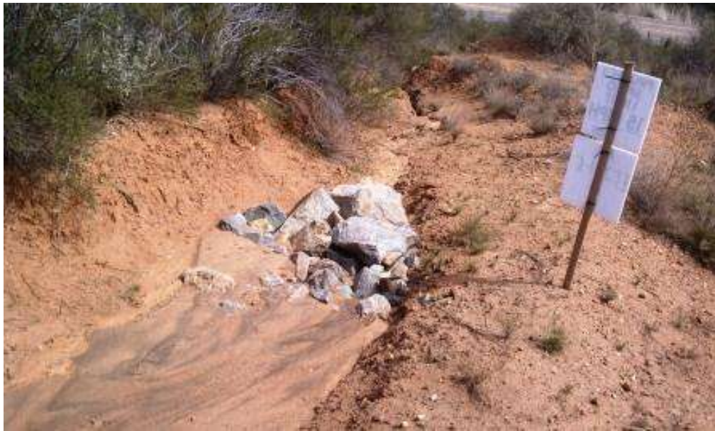
Figure 7: BMPs on access road to Tower CP24 after recent storm. (Link 2)
