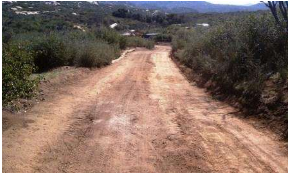
Figure 8: Access road to Tower EP36 after cleanup of hydraulic fluid spill. (Link 2)
