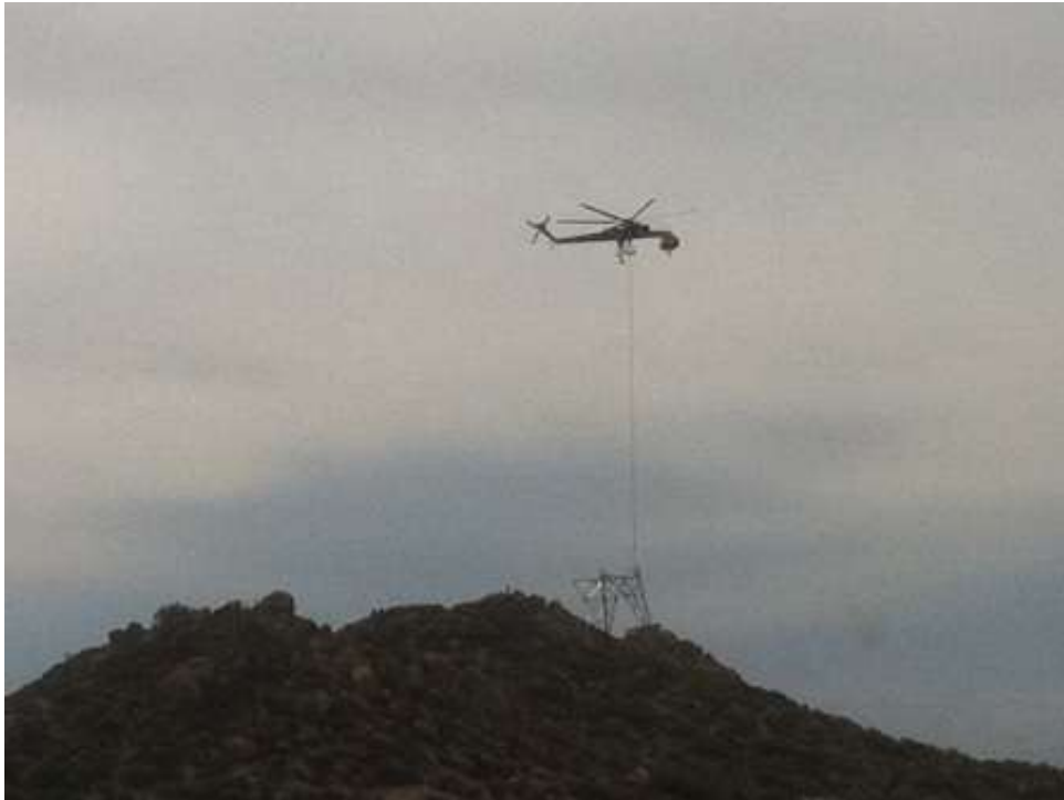
Figure 1: Air crane conducting tower assembly at Tower EP224-1. ( Link 1 )
