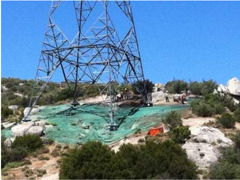
Figure 5: Hydromulching at EP116-3. (Link 2)
