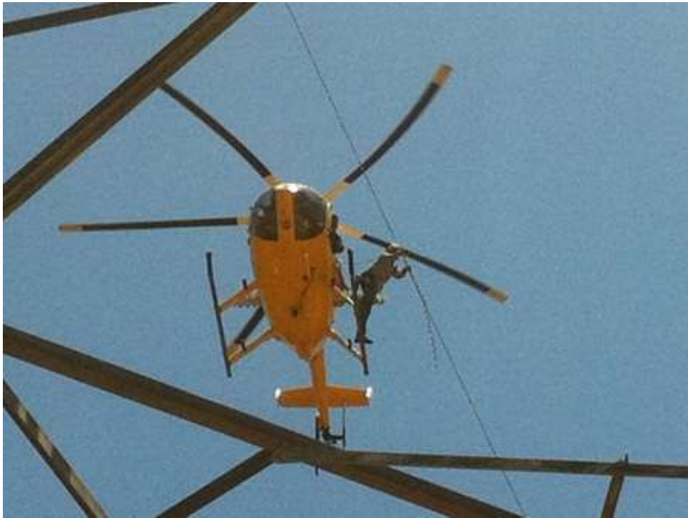
Figure 3: Installing marker balls at EP12-3. (Link 2)
