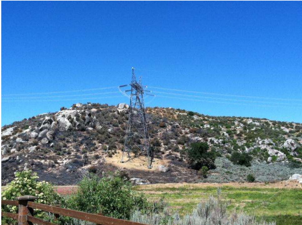
Figure 6: A non-project related fire took place at EP118-2. (Link 2)
