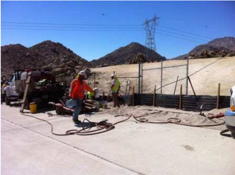
Figure 1: Fence grounding at EP269-1 pull site. (Link 1)
