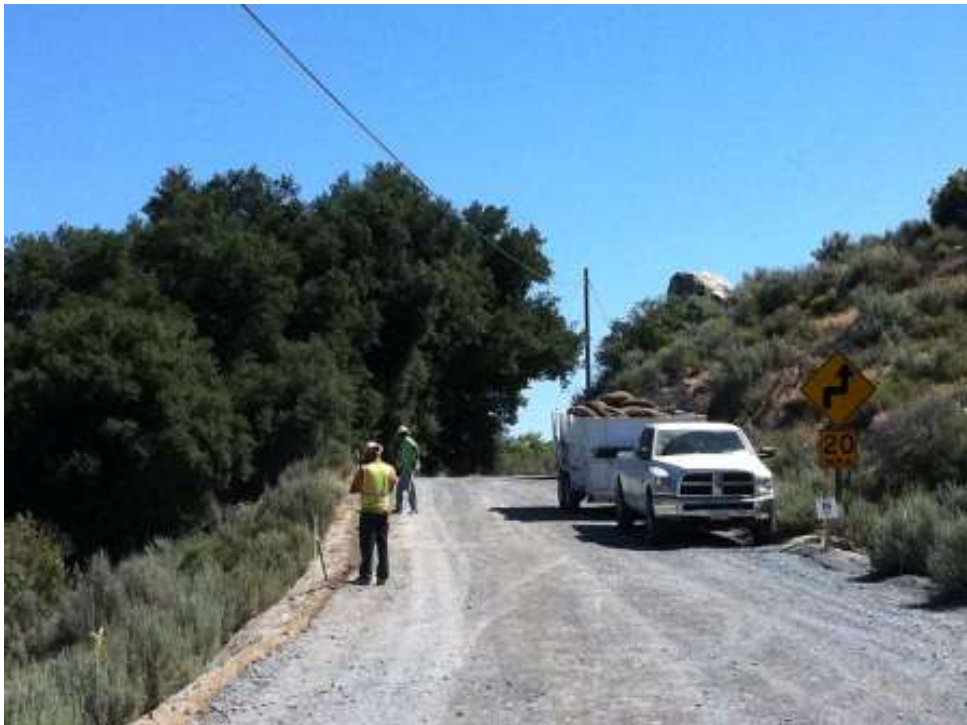
Figure 4: BMP repair work along La Posta Truck Trail. (Link 2)
