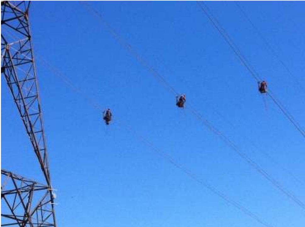
Figure 2: Installing spacers near EP125 pull site. (Link 2)
