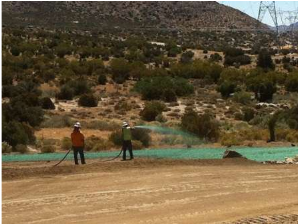
Figure 2: Hydromulching at EP215 pull site. (Link 1)
