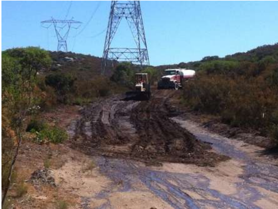
Figure 1: Final road grading near EP96-N-A to EP99-2-N-B. (Link 2)
