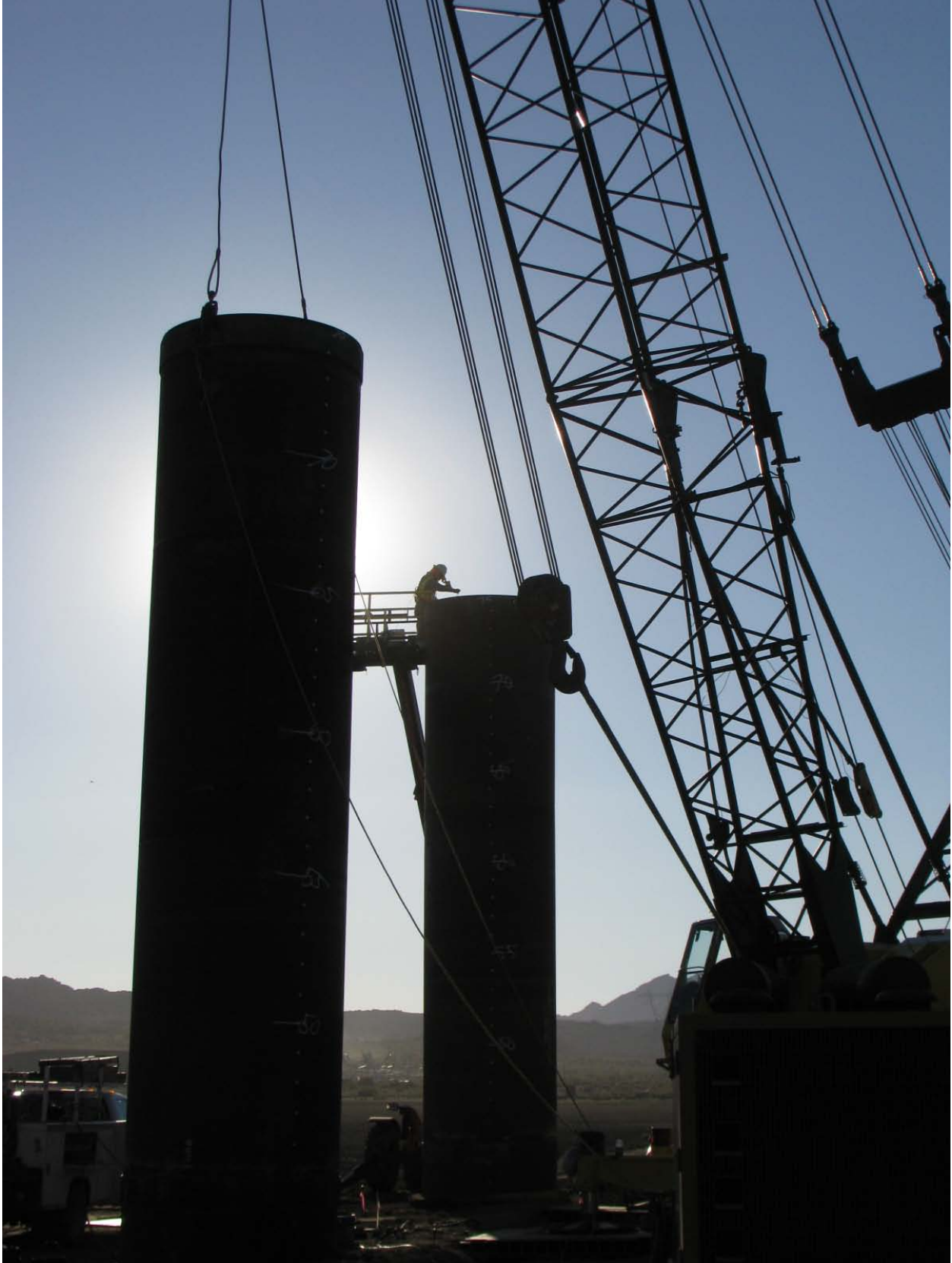
Caisson installation at EP239. Photo courtesy of Erik Strods.
