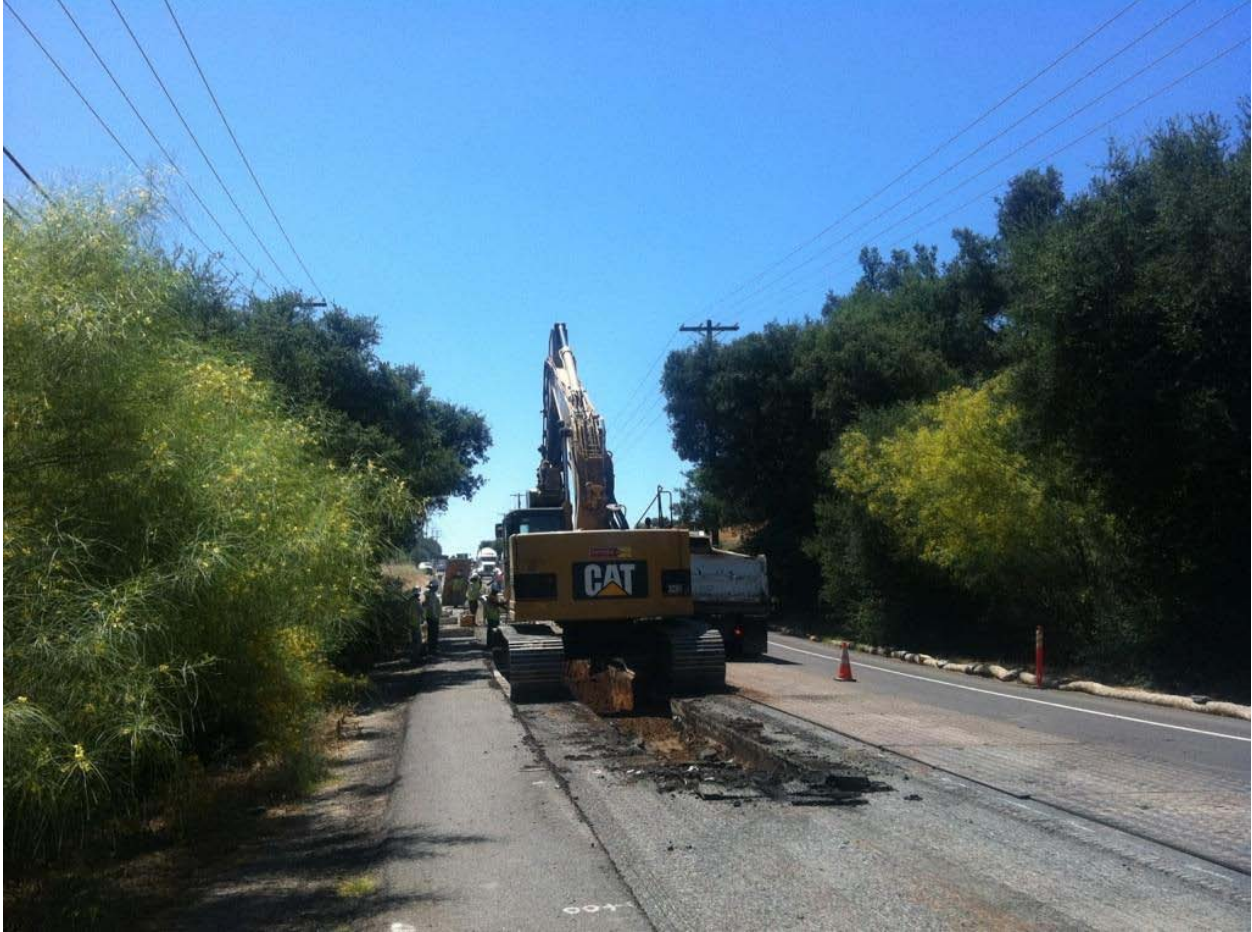
Trenching along Alpine Boulevard. Photo courtesy of Jeff Smith.
