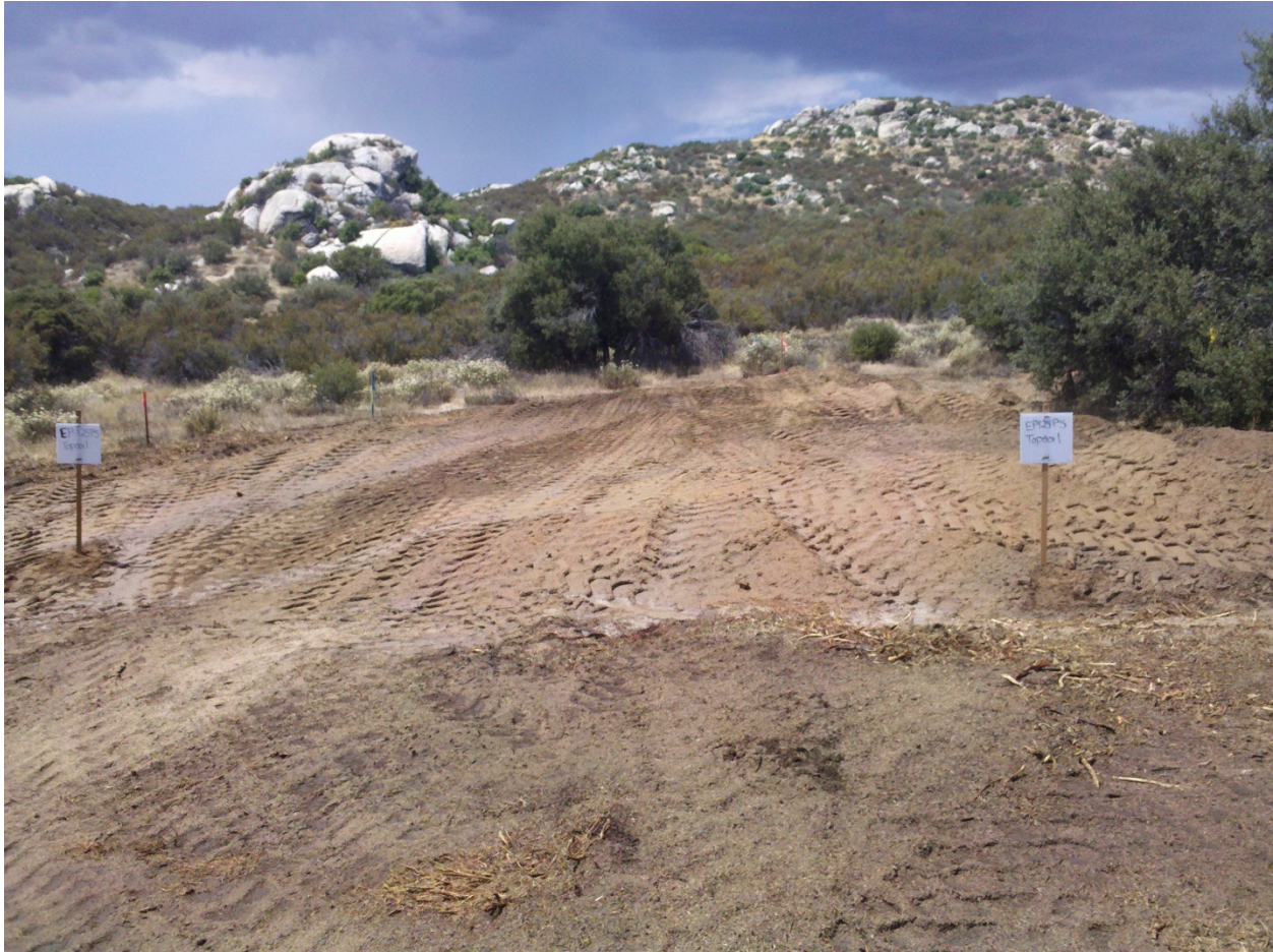
Topsoil salvaging at EP125 pull site. Photo courtesy of Rosina Gallego.
