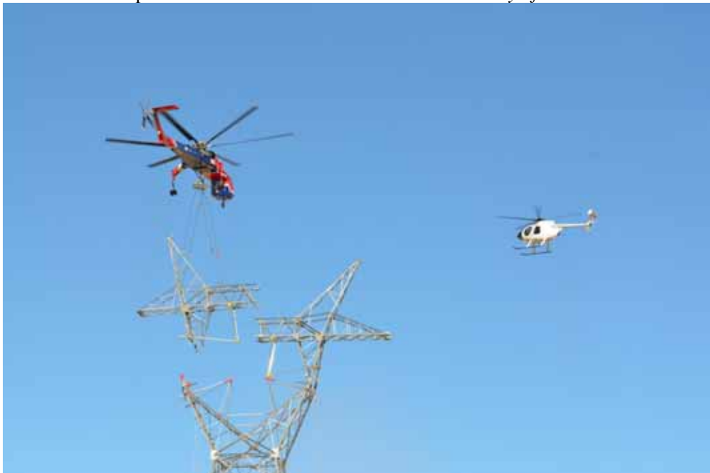
Setting split bridge at EP269. Photo courtesy of Rebecca Carson.
