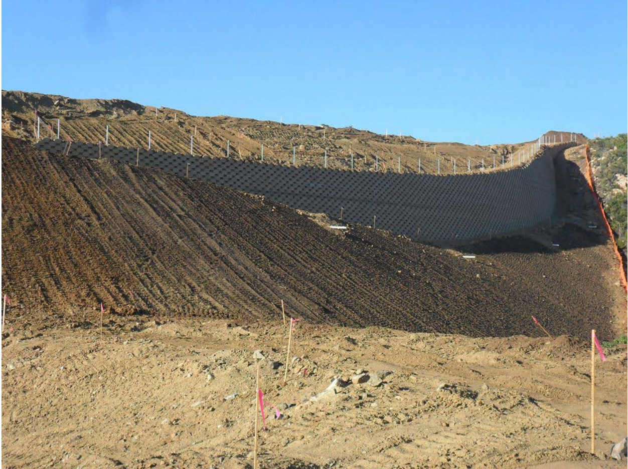
MSE wall at Suncrest Substation. Photo courtesy of Mark Meridith.
