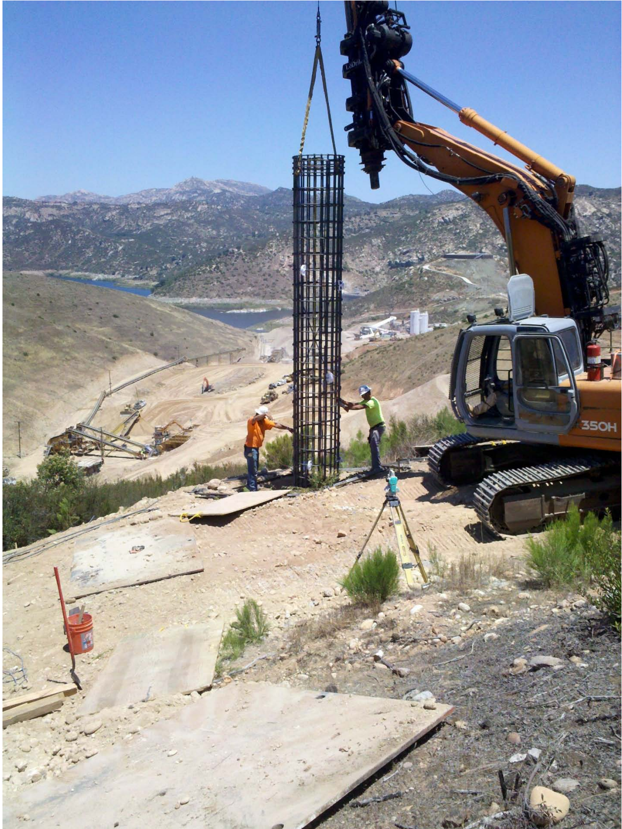
Rebar cage and stub angle set-up. Photo courtesy of Rosina Gallego.
