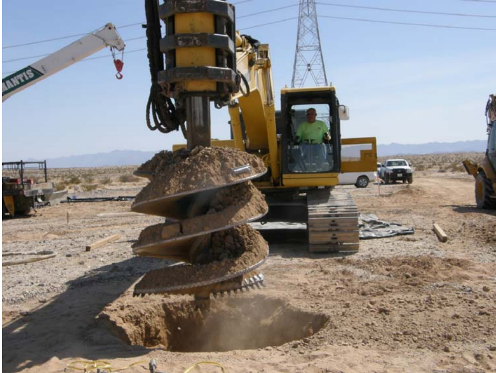
Drilling activities taking place at EP337. Photo courtesy of Don Spires
