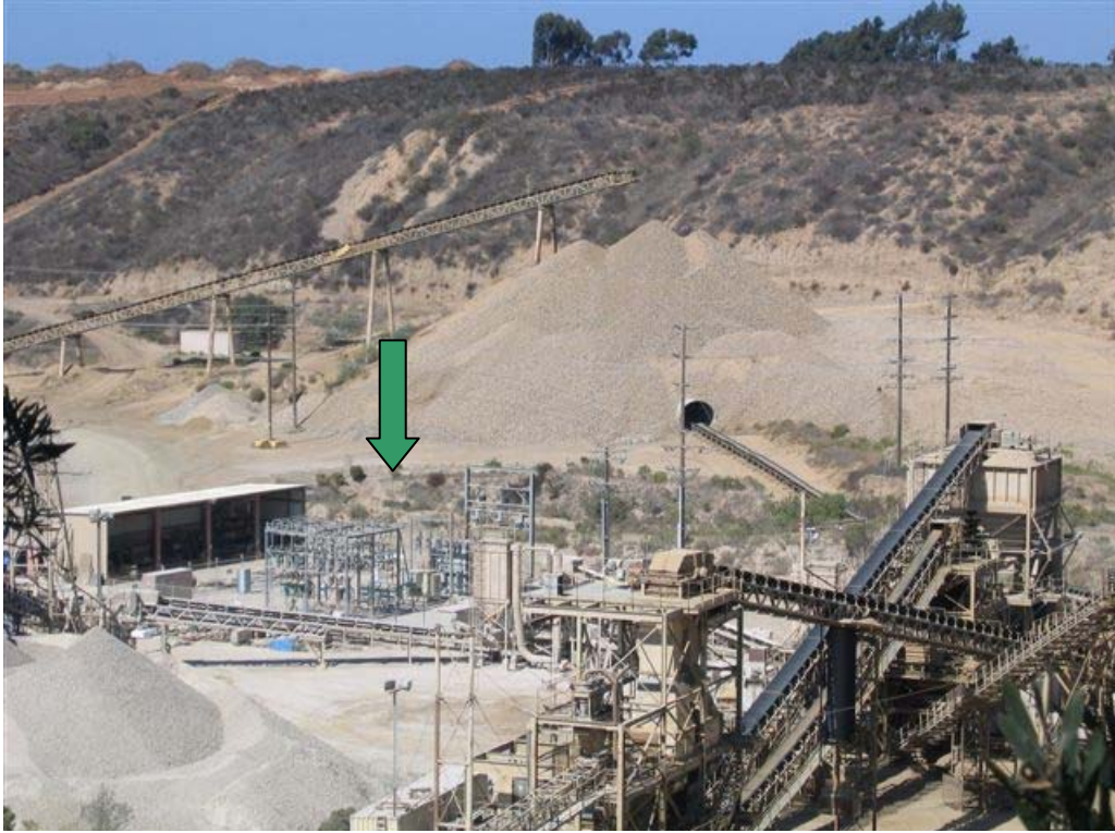
View of rock quarry operation in Fenton Canyon. Fenton substation is below green arrow.
