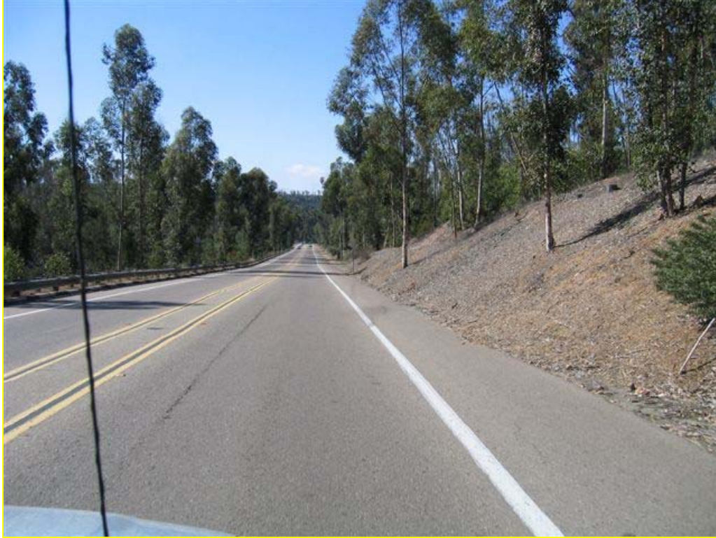
Typical view of Pomerado Road (looking west)
