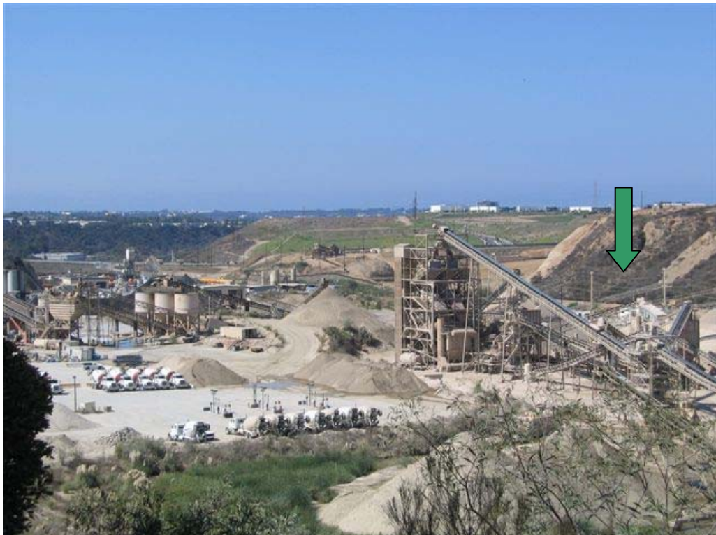
Additional rock quarry operations in Fenton Canyon. Existing 69 kv lines are below green arrow.
