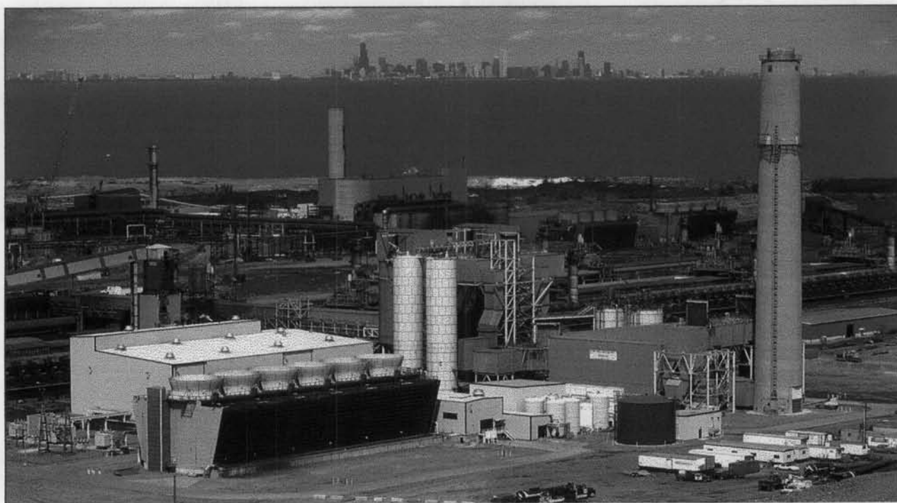
Figure 1. Cokerenergy – Energy Recycling Plant at Mittal Steel, East Chicago, Indiana
