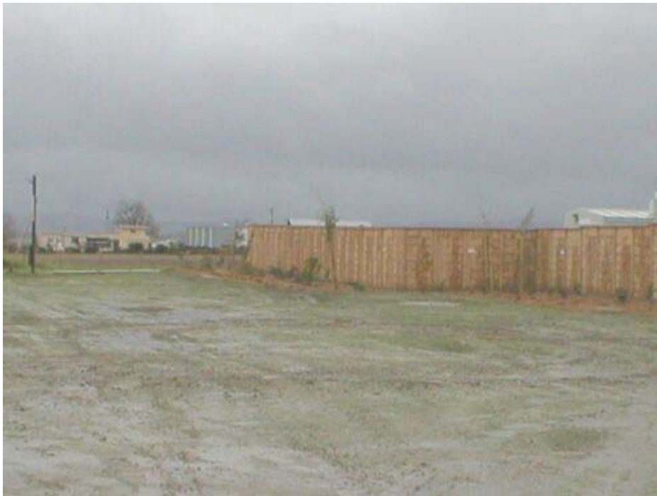
Figure 5 – Cayetano Substation, note vegetation and rutted foreground area, Phase Two.
