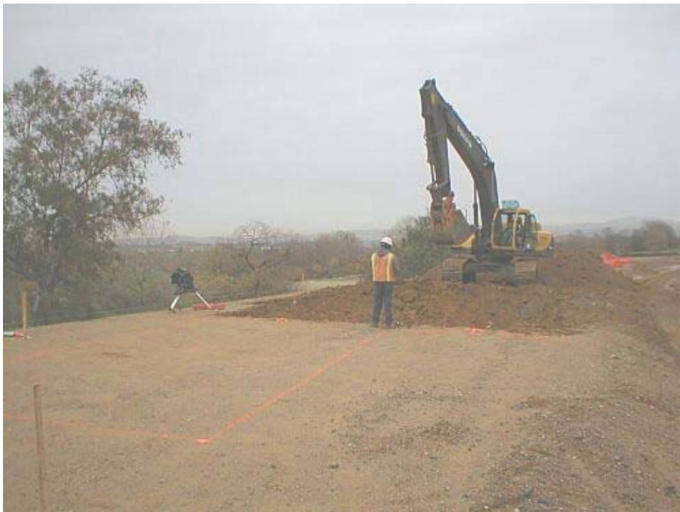
Figure 3 Vault 14A and 14B excavation along New Vineyard Road.
