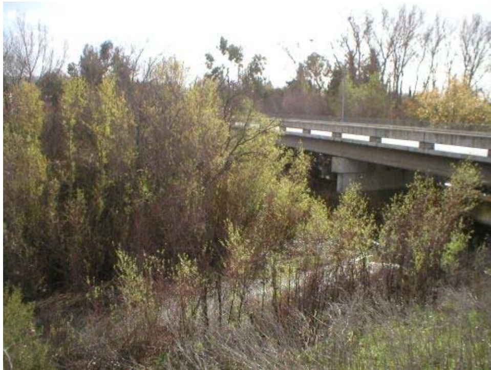
Figure 1 Arroyo del Valle crossing at Bernal Avenue (bore location).
