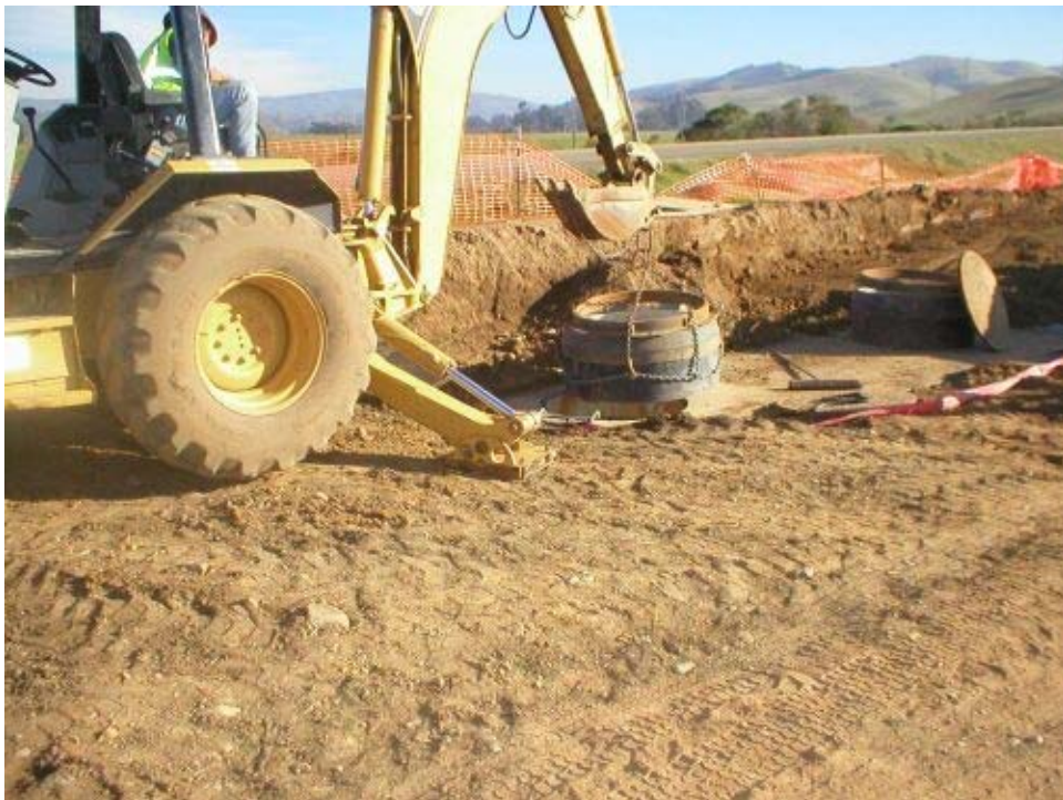
Figure 4 Vault 3A and 3B construction.
