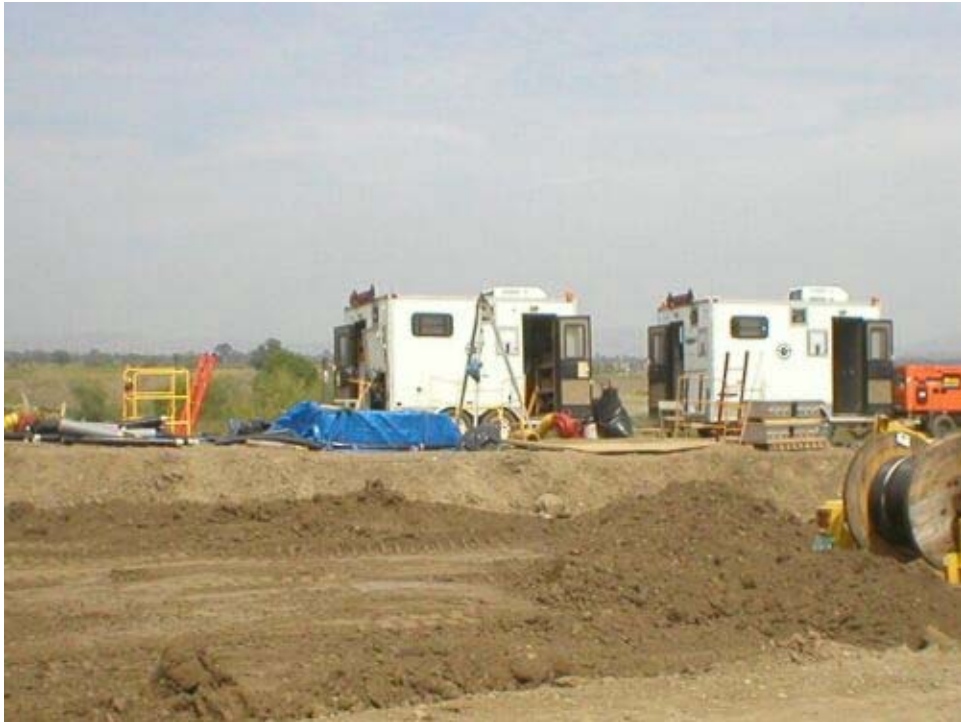
Figure 2 – Splicing at the Vault 12 location along New Vineyard Road.
