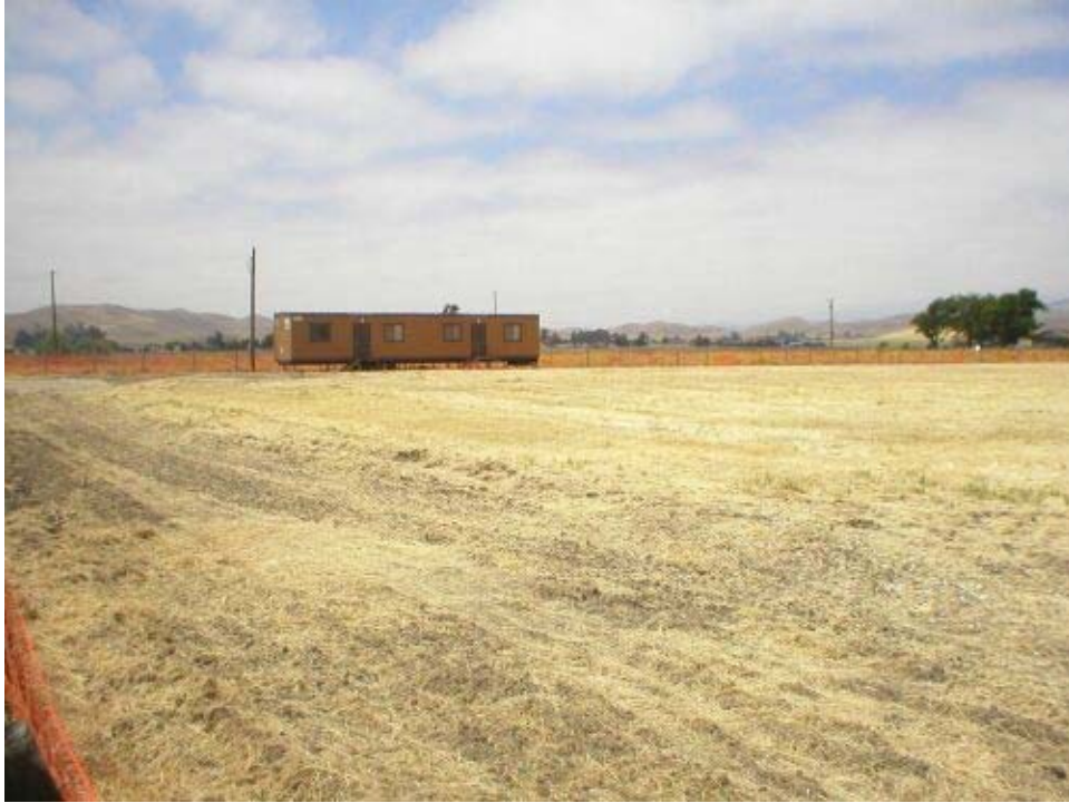
Figure 3 – PSD Contractor Yard, A trailer has been placed within the yard and a power pole installed, Phase Two.
