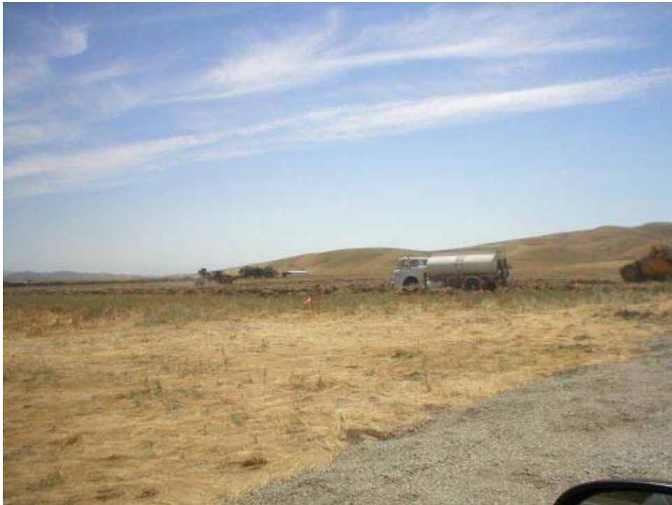
Figure 2 – Grading at the Cayetano Substation Area, Phase Two.
