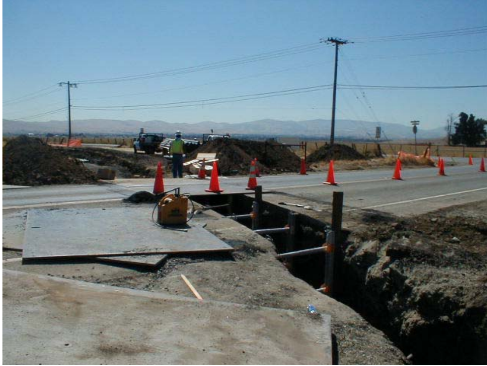
Figure 1 – Trenching and conduit installation across North Livermore Avenue, Phase Two.
