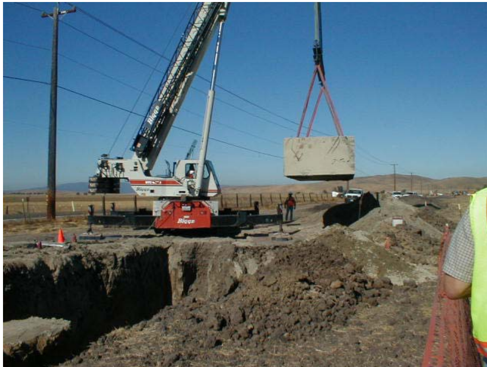
Figure 2 – Replacement of a damaged vault along May School Road, Phase Two.
