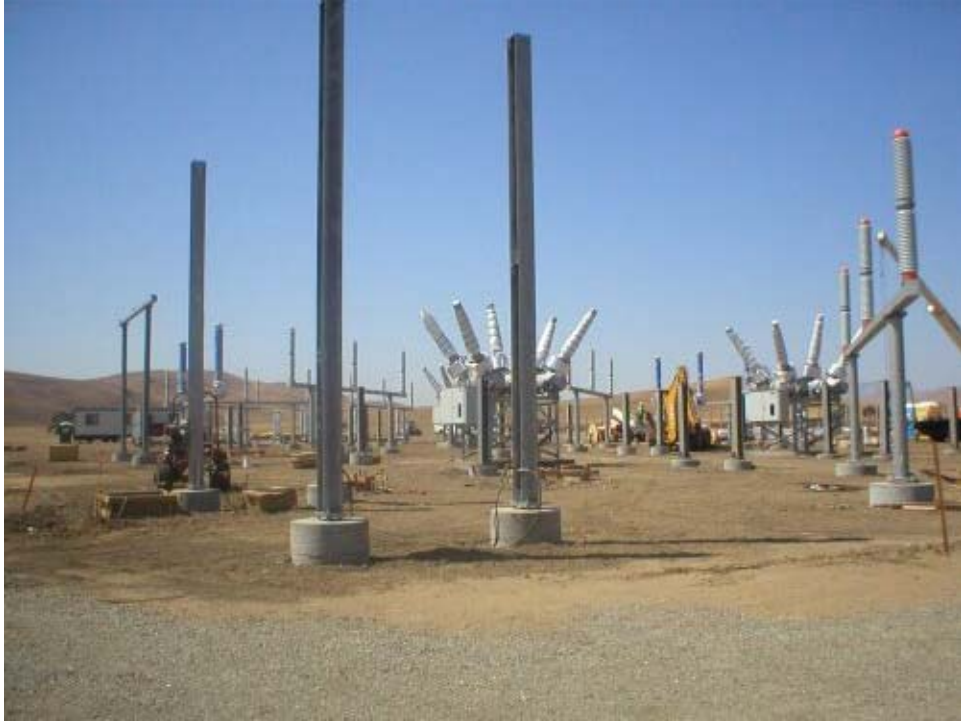
Figure 1 – Substation component installation, Cayetano Substation, Phase Two.
