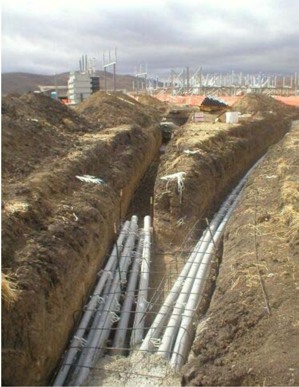
Figure 2 – Conduit installation leading to the Cayetano Substation, Phase Two.
