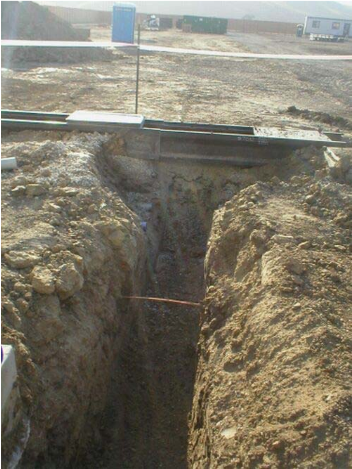
Figure 1 - Un-ramped trench at the Cayetano Substation, Phase Two.
