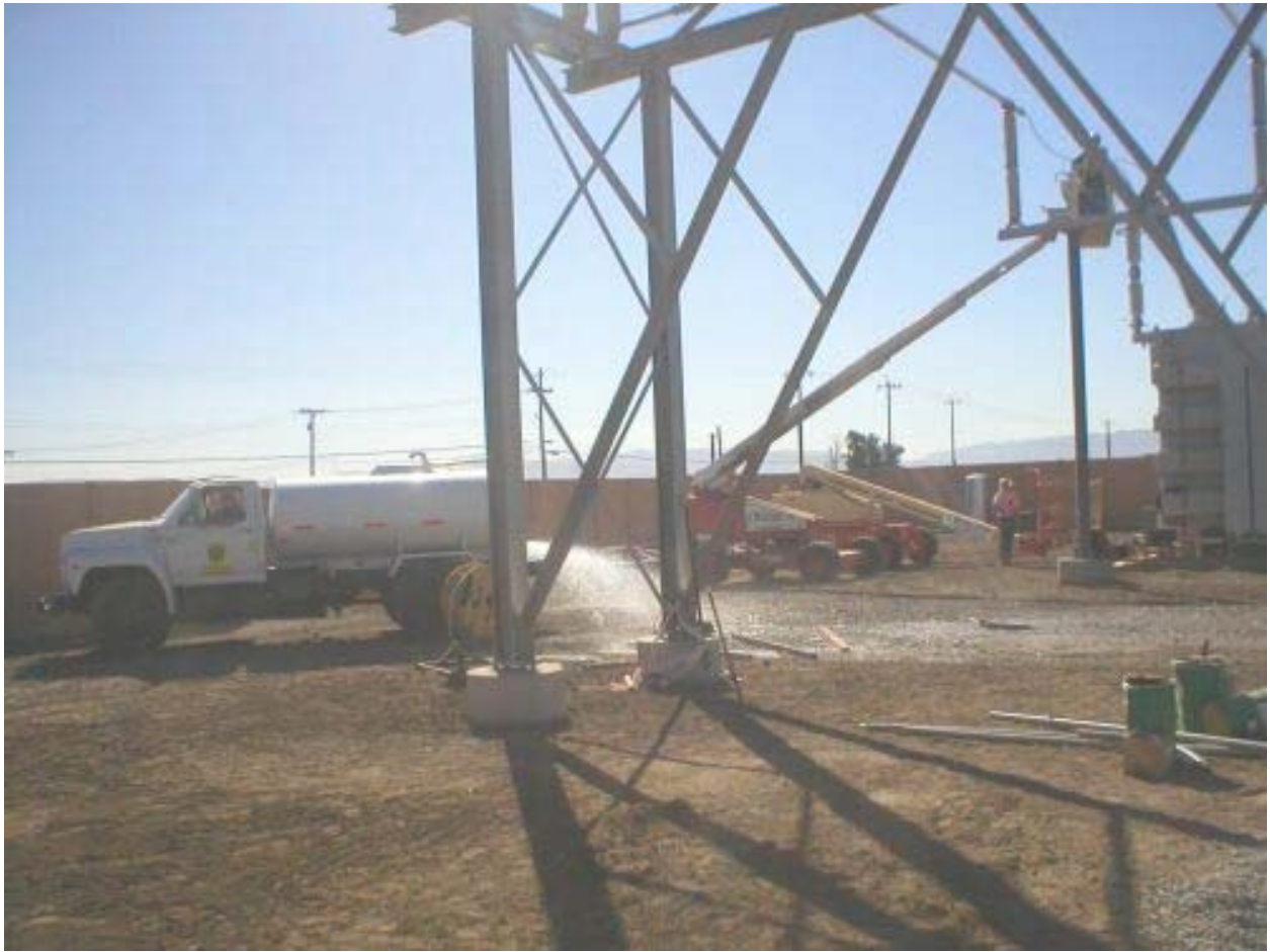
Figure 1 – Watering to suppress dust at the Cayetano Substation, Phase Two.
