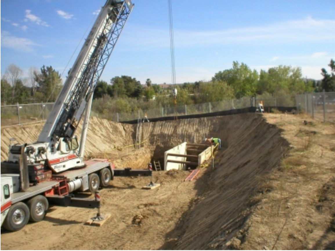
Figure 1: Arroyo Del Valle north bore pit shoring placement.
