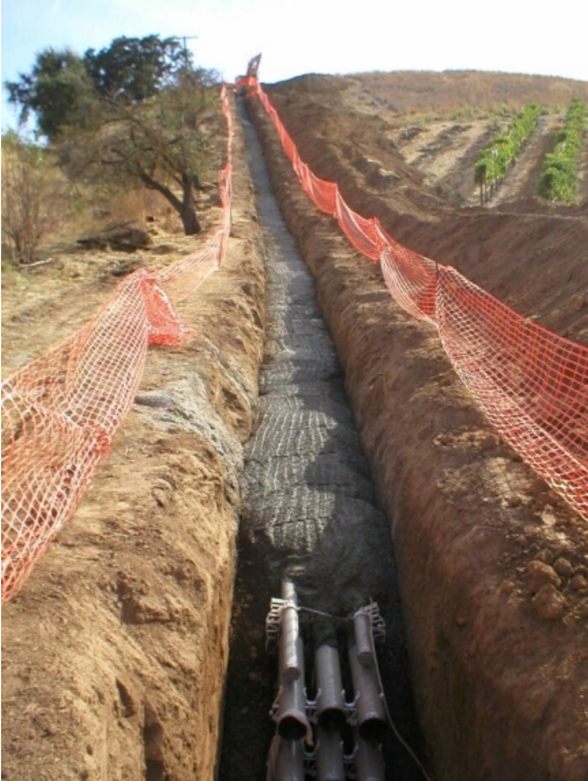
Figure 2: Trenching and conduit installation at Station 26+50 working down a steep slope.
