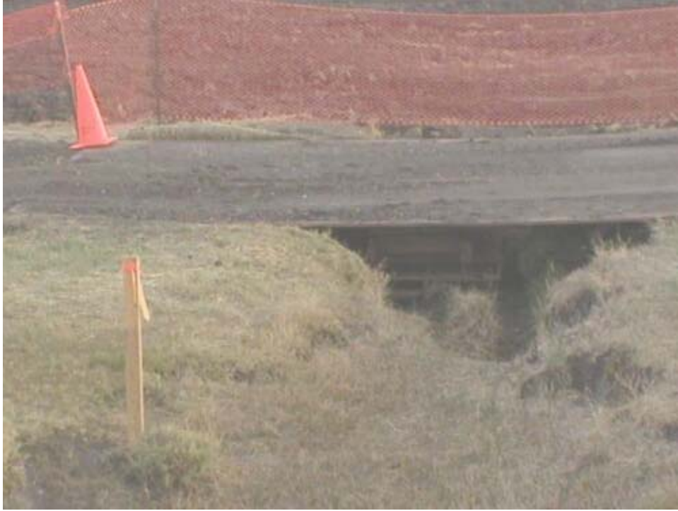
Figure 4 – Pallets placed in the USACE drainage along the access road leading to the Transition Station, Phase Two.
