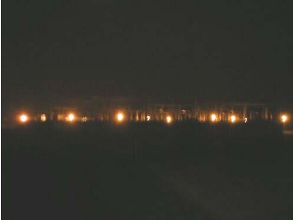
Figure 2 – Night lighting at the Cayetano Substation., Phase Two.
