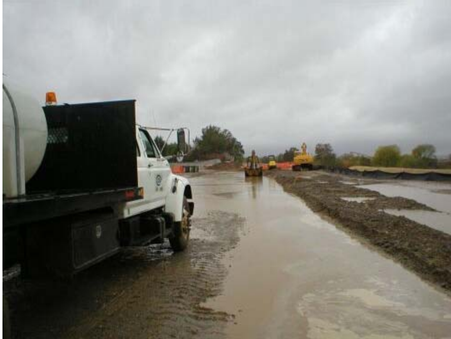
Figure 1 New Vineyard Road Flooding on November 8 th .
