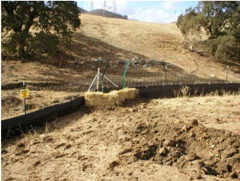
Figure 4 Added erosion control device installation at the Transition Station site.
