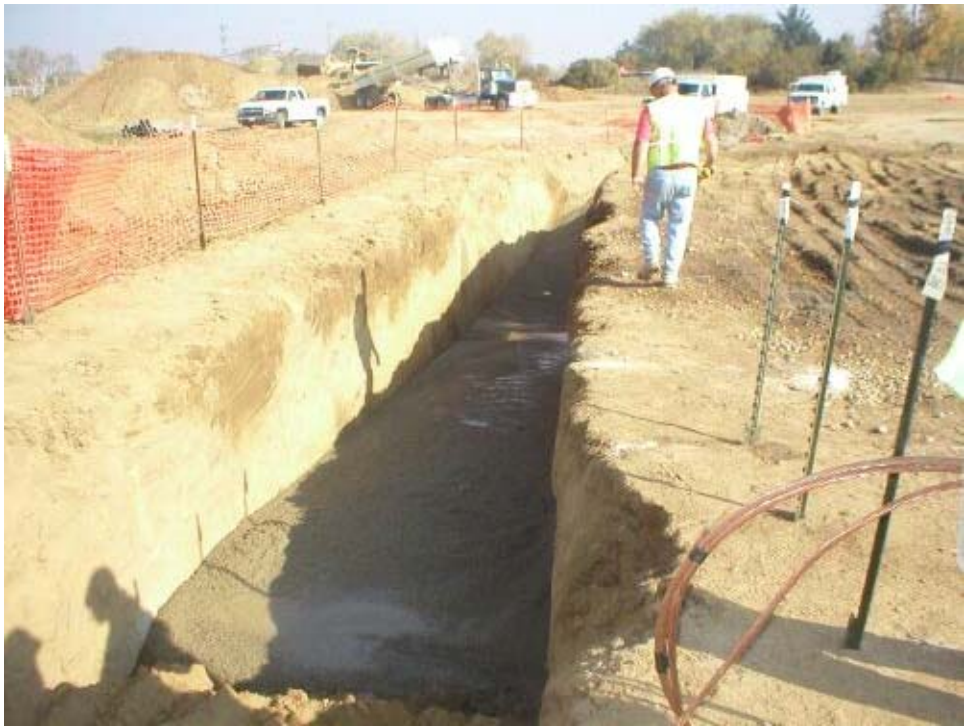
Figure 1 Fresh concrete within the trench line extending from the Vineyard Substation.
