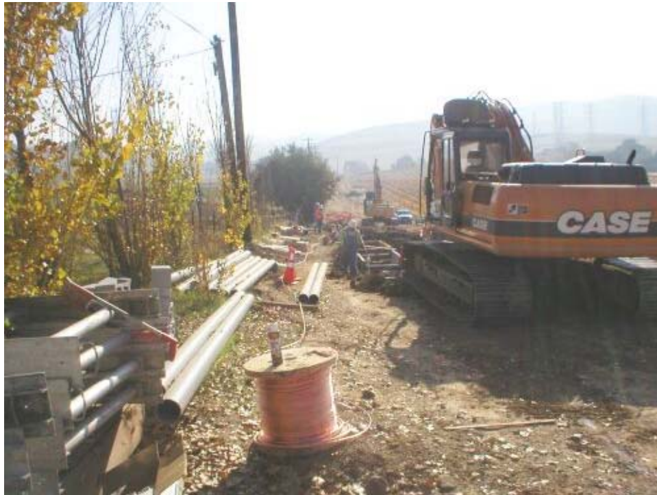
Figure 3 Trenching under a waterline west of the Transition Station site.
