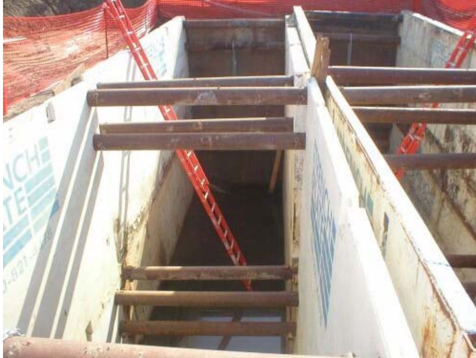
Figure 2 Shoring installed within the Arroyo del Valle north bore pit.
