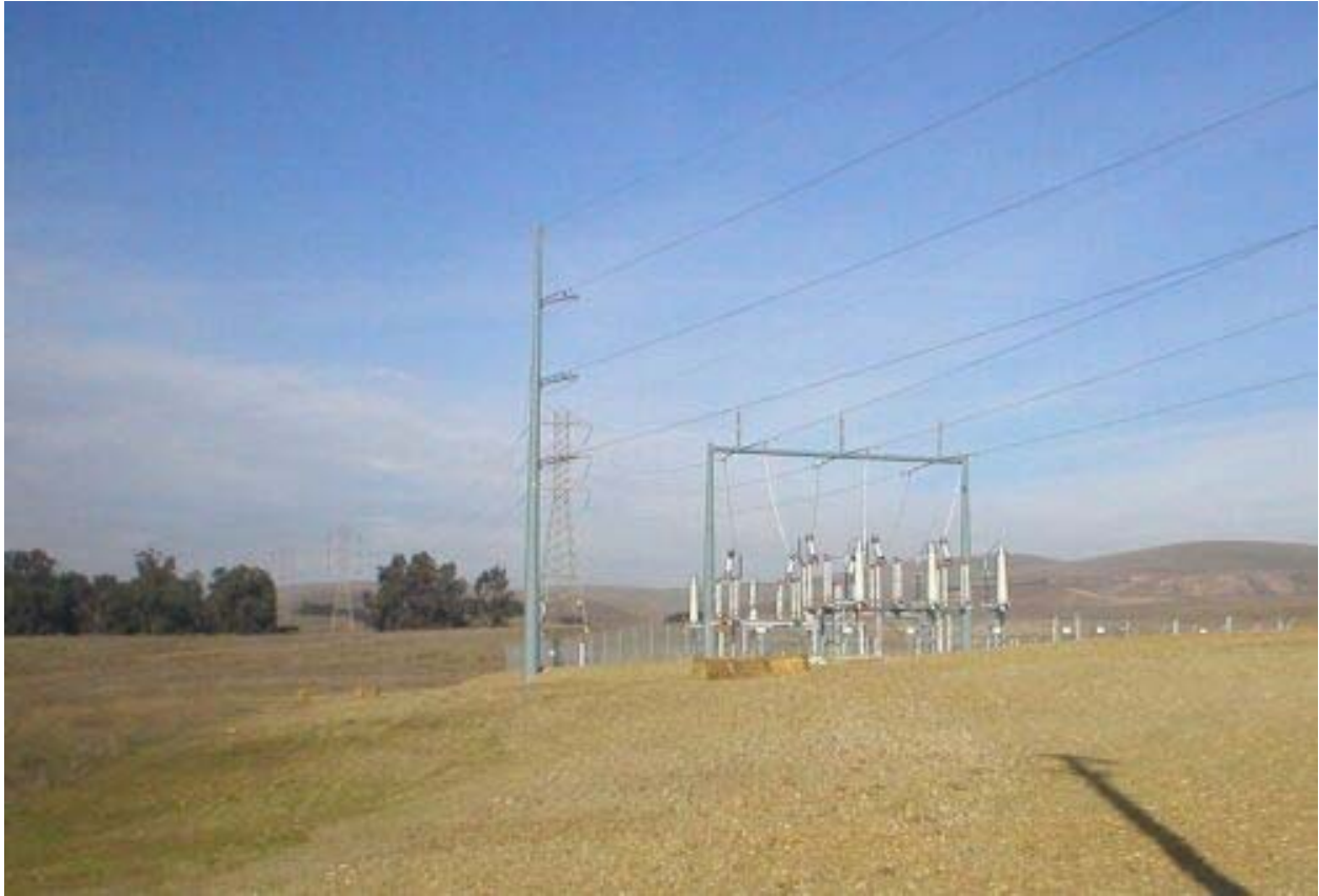
Figure 2 – Hay bales have installed for added erosion control around the previously hydro-seeded area surrounding the Transition Station, Phase Two
