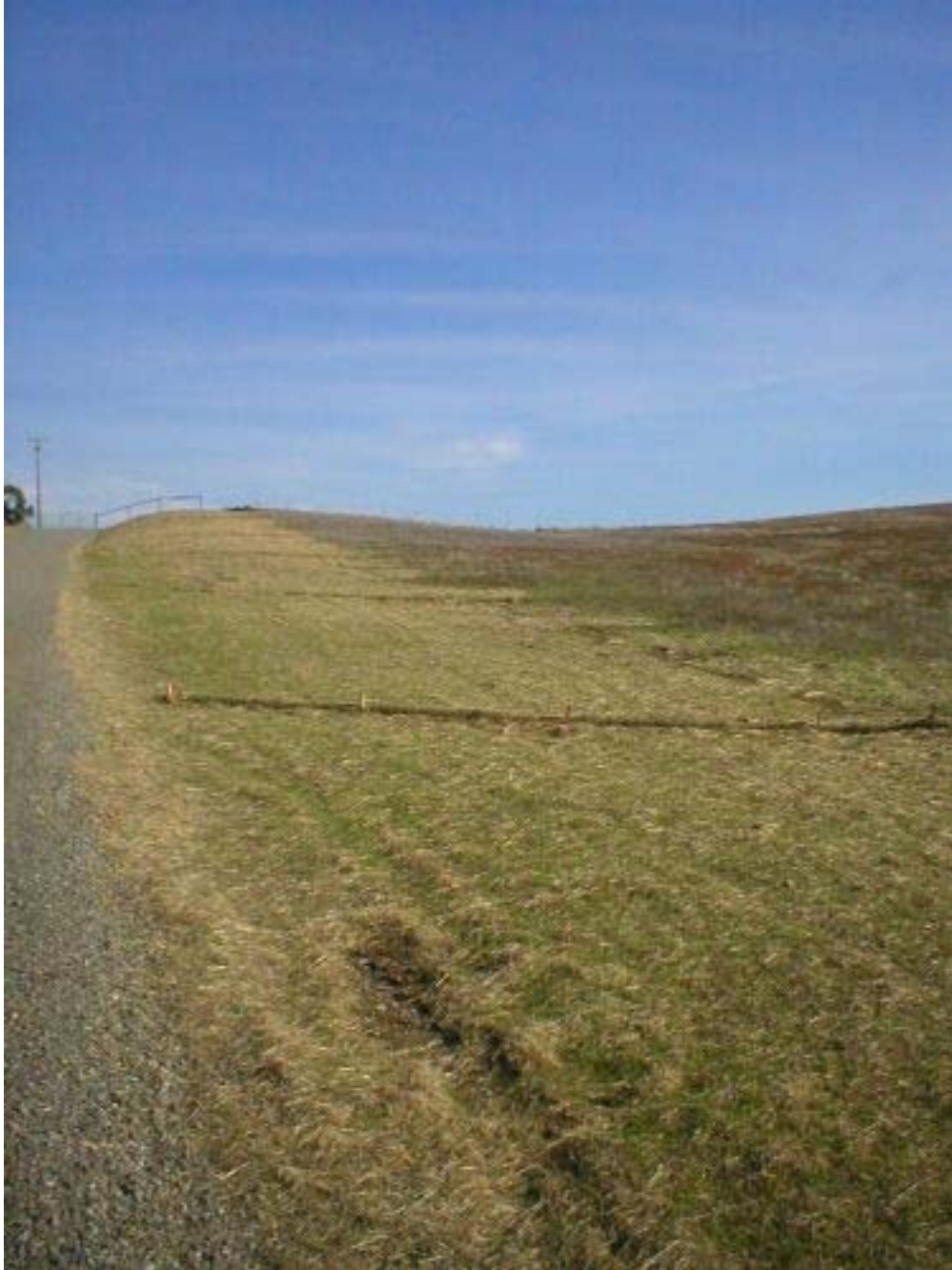
Figure 1 – Straw waddle waterbars have been installed and staked along the previously hydro-seeded steep slope along the access road leading to the Transition Station, Phase Two
