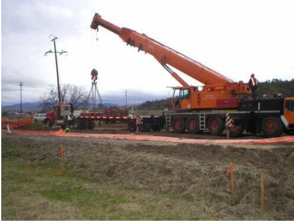
Figure 1 Vault installation along New Vineyard Road.
