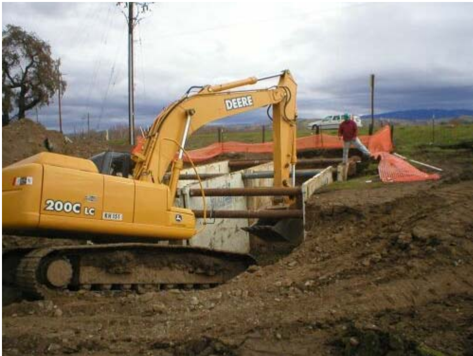
Figure 2 Shoring installation within the western pit of the Highway 84 bore.
