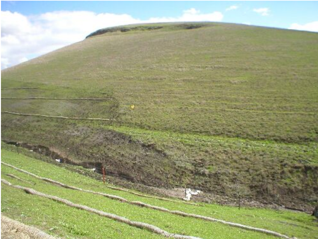
Figure 2 – Incised drainage along the underground alignment, March 6, 2006.
