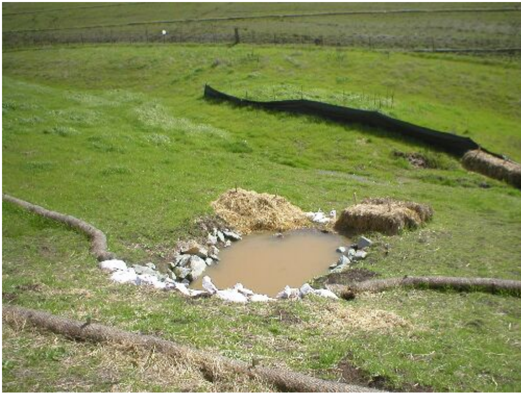
Figure 3 – Culvert outlet along Road 7, March 6, 2006.
