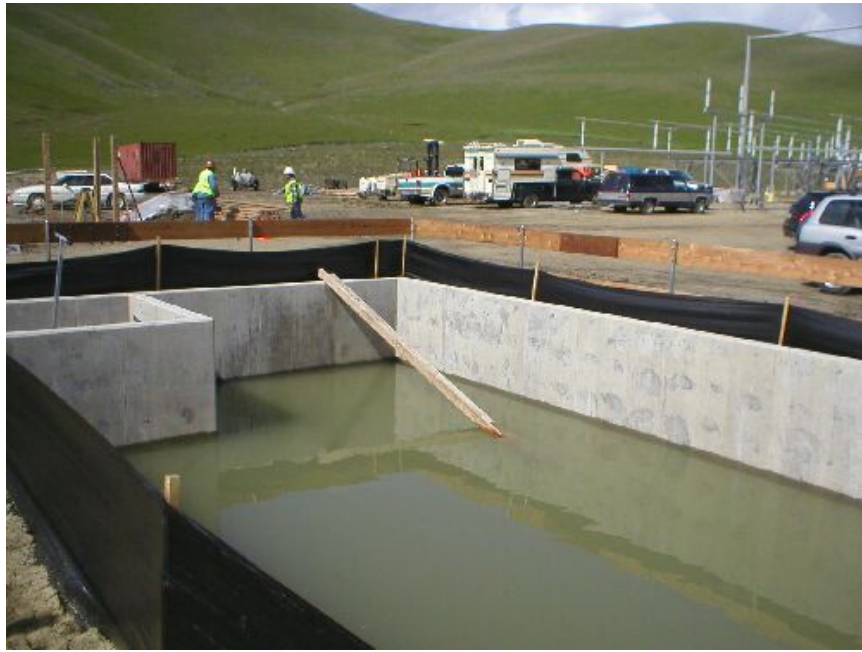
Figure 3 – SPCC pond with sediment fence installed around the perimeter, March 15, 2006.
