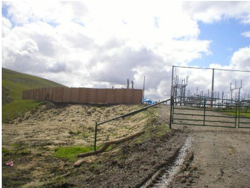
Figure 2 – Concrete wall installed around the North Dublin Substation, March 15, 2006.
