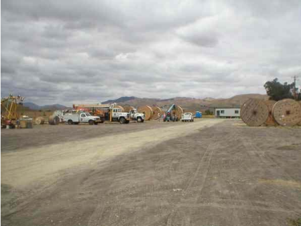
Figure 1 – Wilson yard. Note the transmission cable reels and pulling equipment. June 13, 2006.
