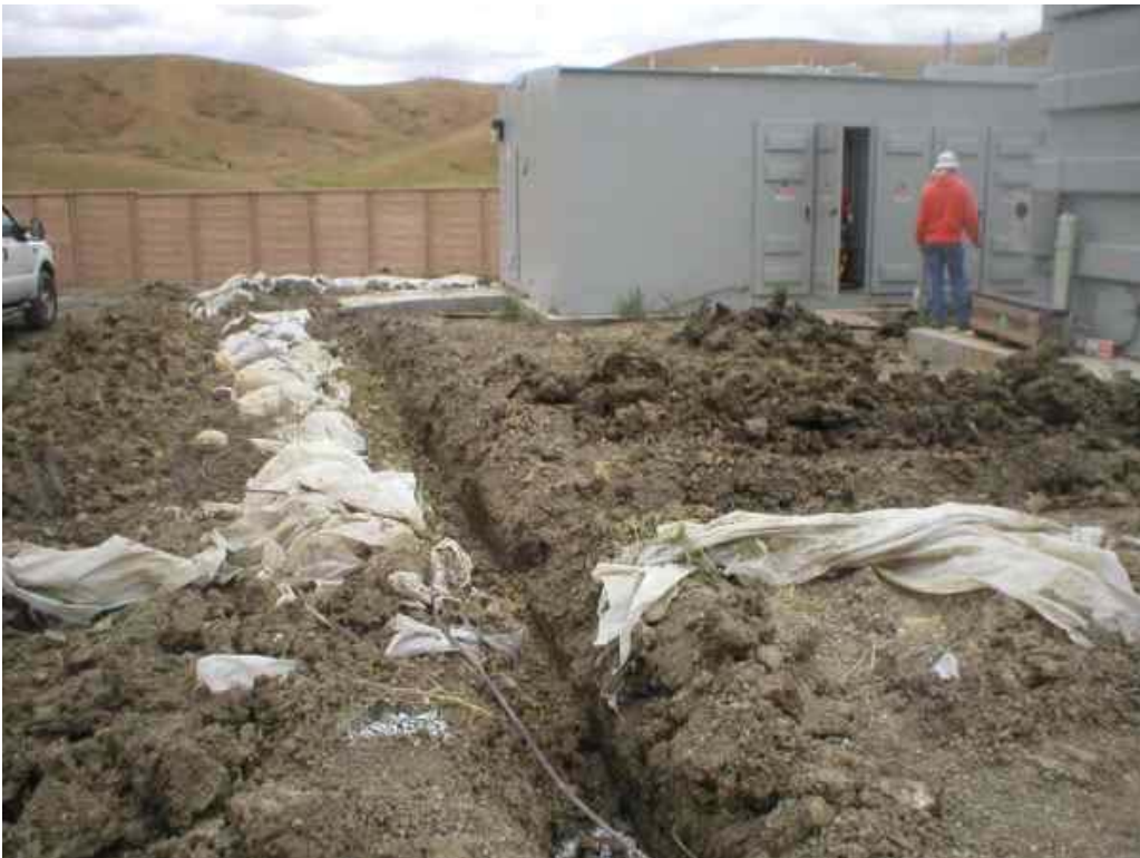
Figure 2 – Trench for the grounding grid at the North Dublin Substation. June 13, 2006.
