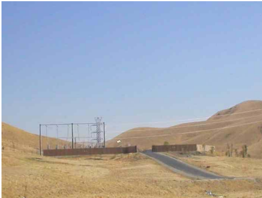
Figure 5 – Drops were installed at the North Dublin Substation, August 18, 2006.
