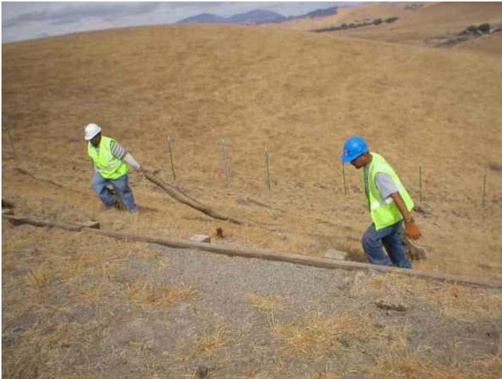
Figure 3 – NVC crews removing wattles downslope of the Transition Station, October 4, 2006.
