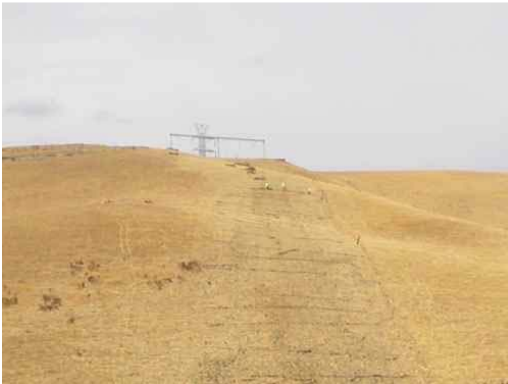
Figure 4 – Crews removing wattles downslope of the Transition Station, October 4, 2006.
