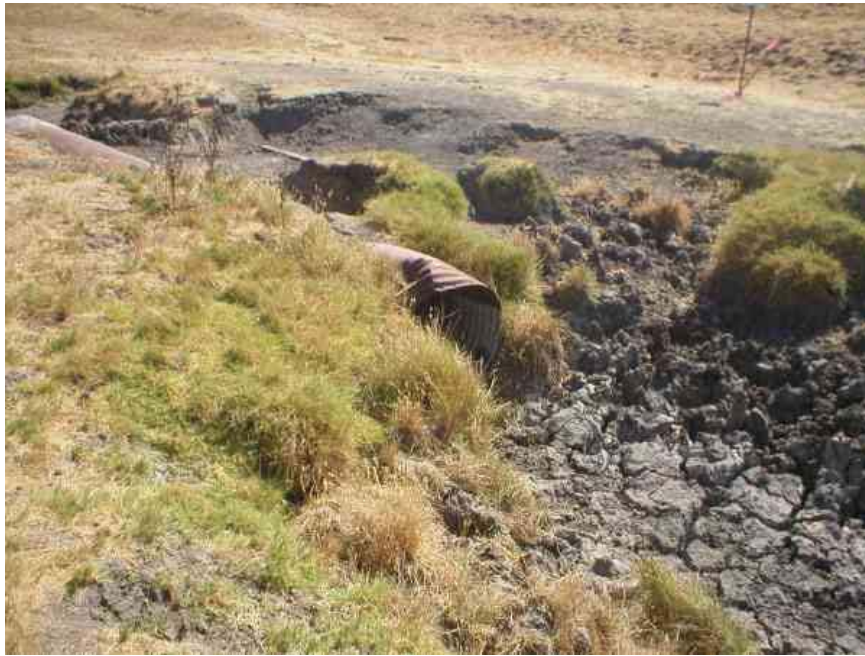
Figure 3 – Culvert within the jurisdictional waterway which is slated for replacement, August 24, 2006.
