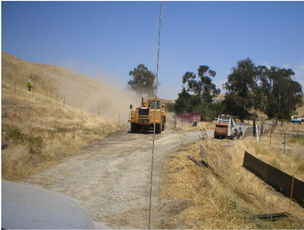
Figure 2 – Dust produced by grading operations, Phase Three, July 15, 2005.
