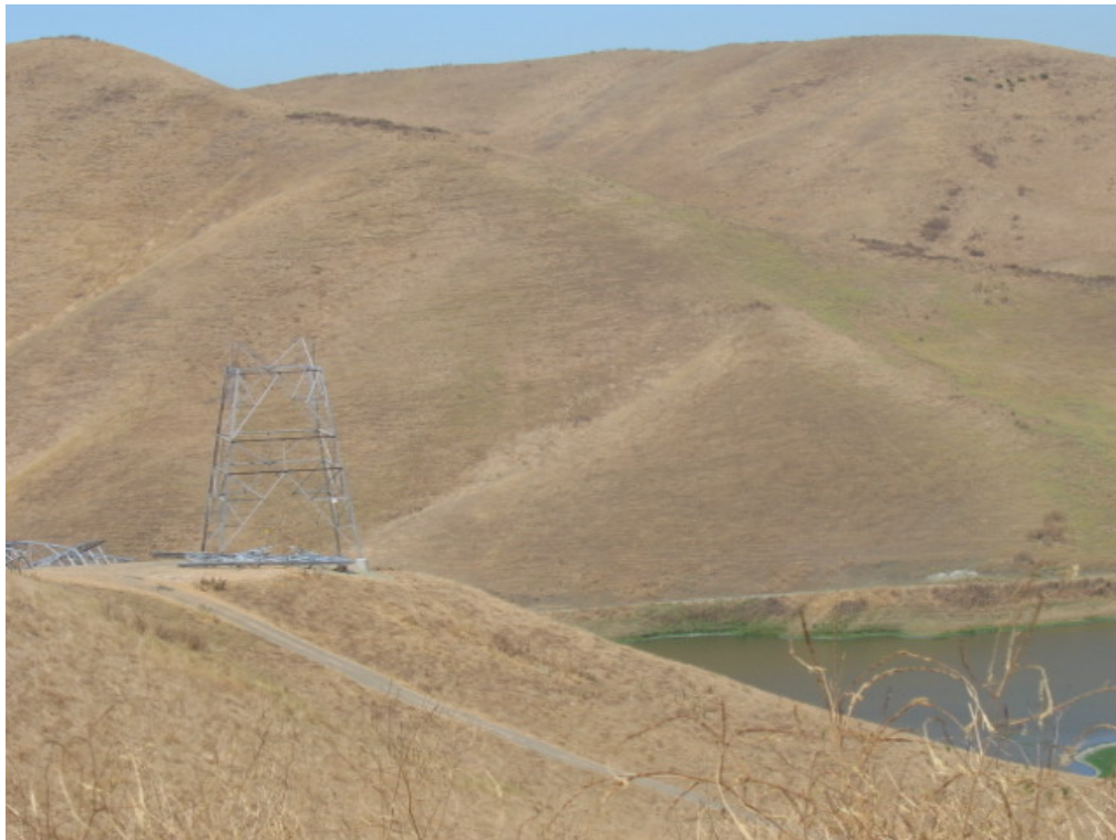
Figure 2 – Construction of Tower 7, August 3, 2005.
