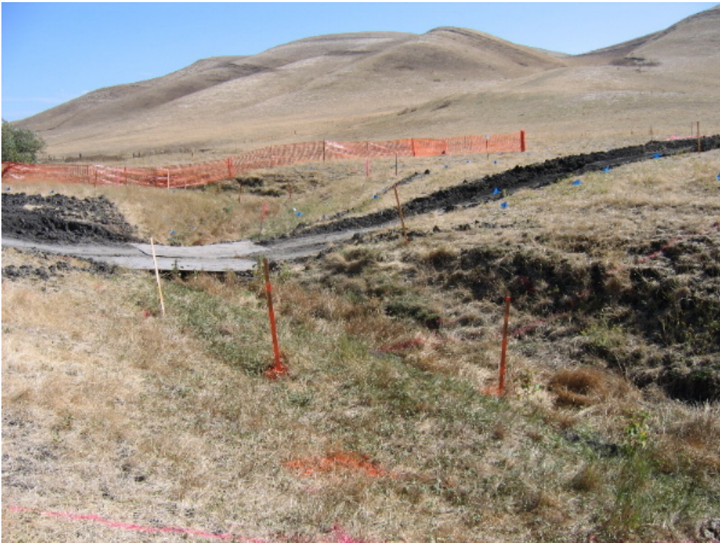
Figure 2 – Cayetano Creek crossing of Access Road 6 before permanent culvert installation, September 22, 2005.
