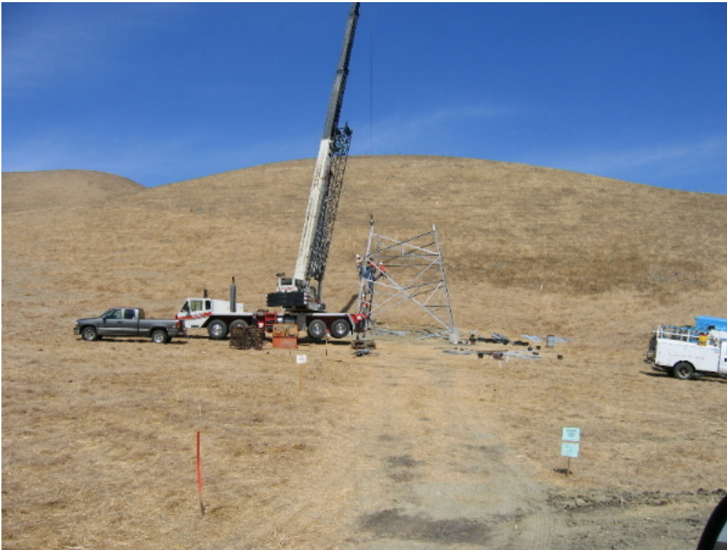
Figure 4 – Tower 1 construction near Moller Road, September 21, 2005.
