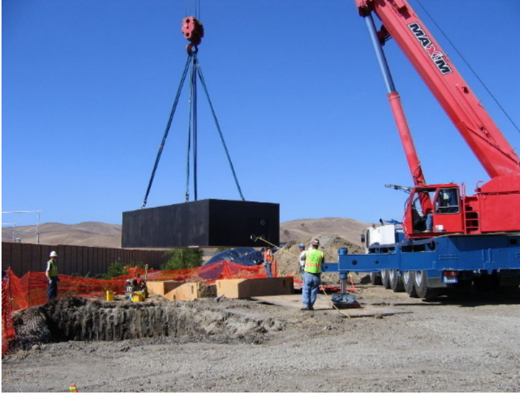
Figure 1 – Vault installation near the North Livermore Substation, September 23, 2005.
