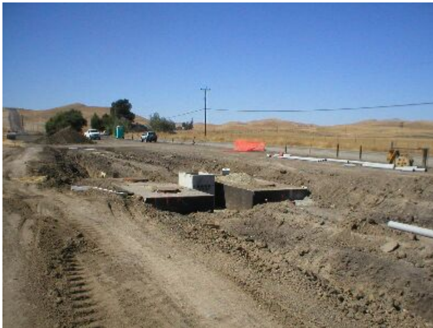
Figure 2 – Vault installation north of the Cayetano Substation, October 5, 2005.
