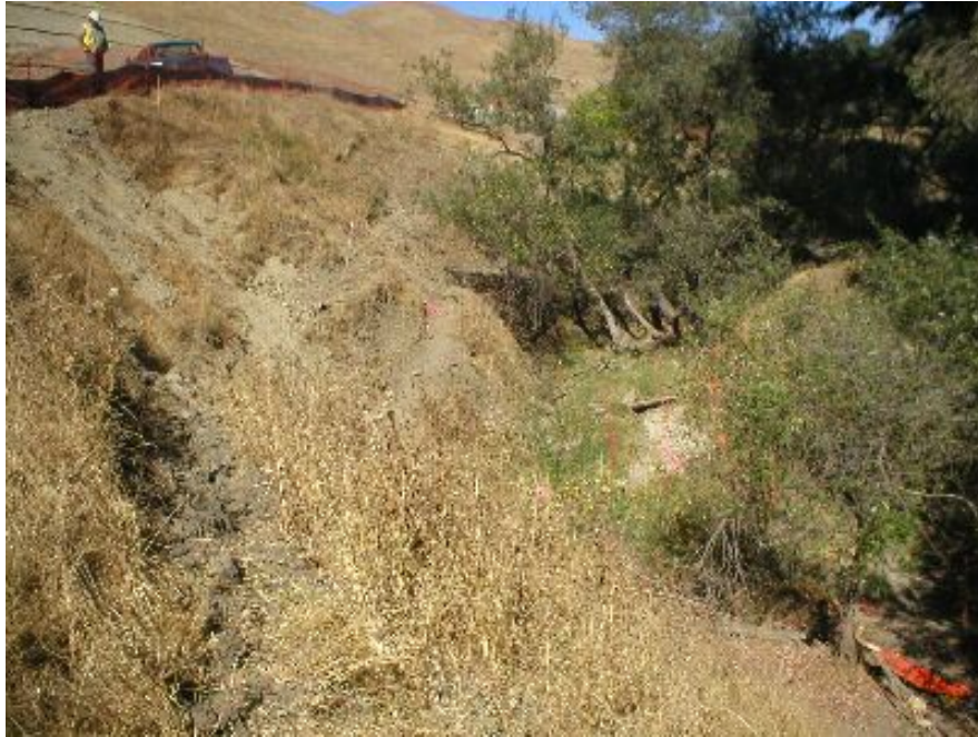
Figure 1 – Bank stabilization area within Tassajara Creek, October 4, 2005.
