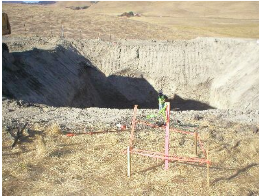
Figure 4 – Vault excavation at the transition station, October 5, 2005.
