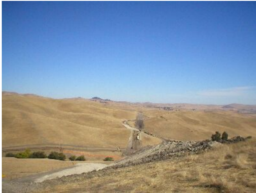
Figure 3 – Road 7 and underground alignment, October 5, 2005.
