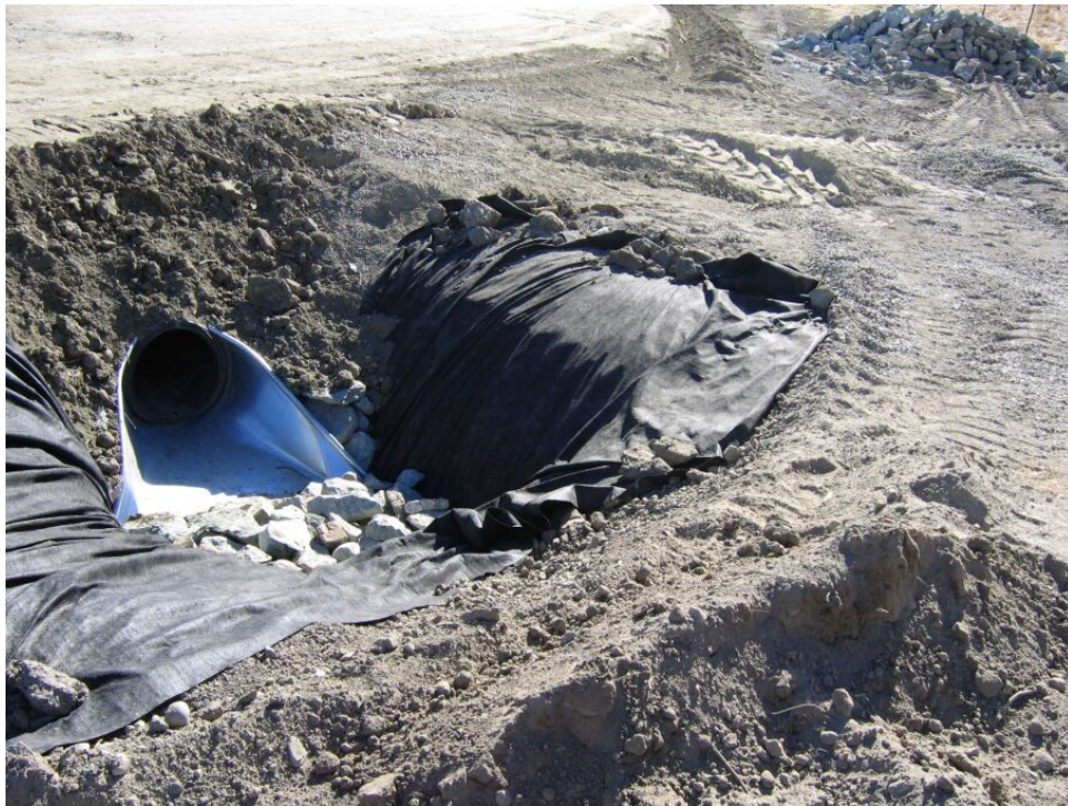
Figure 2 – Culvert installation along Moller Ranch Road, October 12, 2005.
