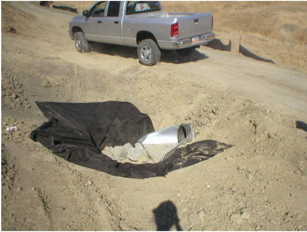
Figure 3 – Culvert undergoing installation along Moller Ranch Road.
